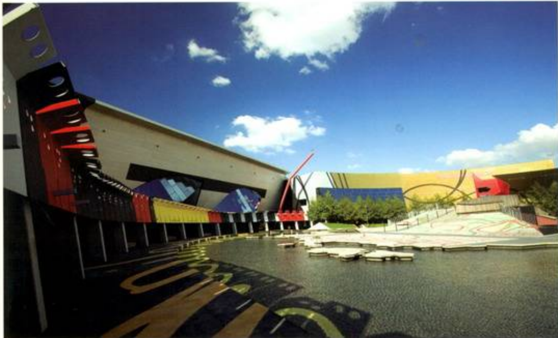
National Museum of Australia, ACT, air conditioning and mechanical services by Environ in 1997
