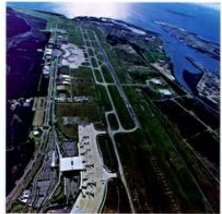
Brisbane Airport air conditioning by Haden Engineering
