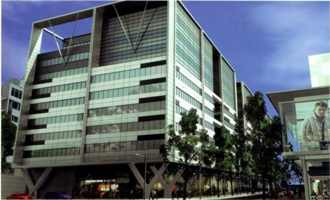
Haden's largest & most complex design and construct project underway, The Australian Tax Office, Precinct C & B, ACT.
