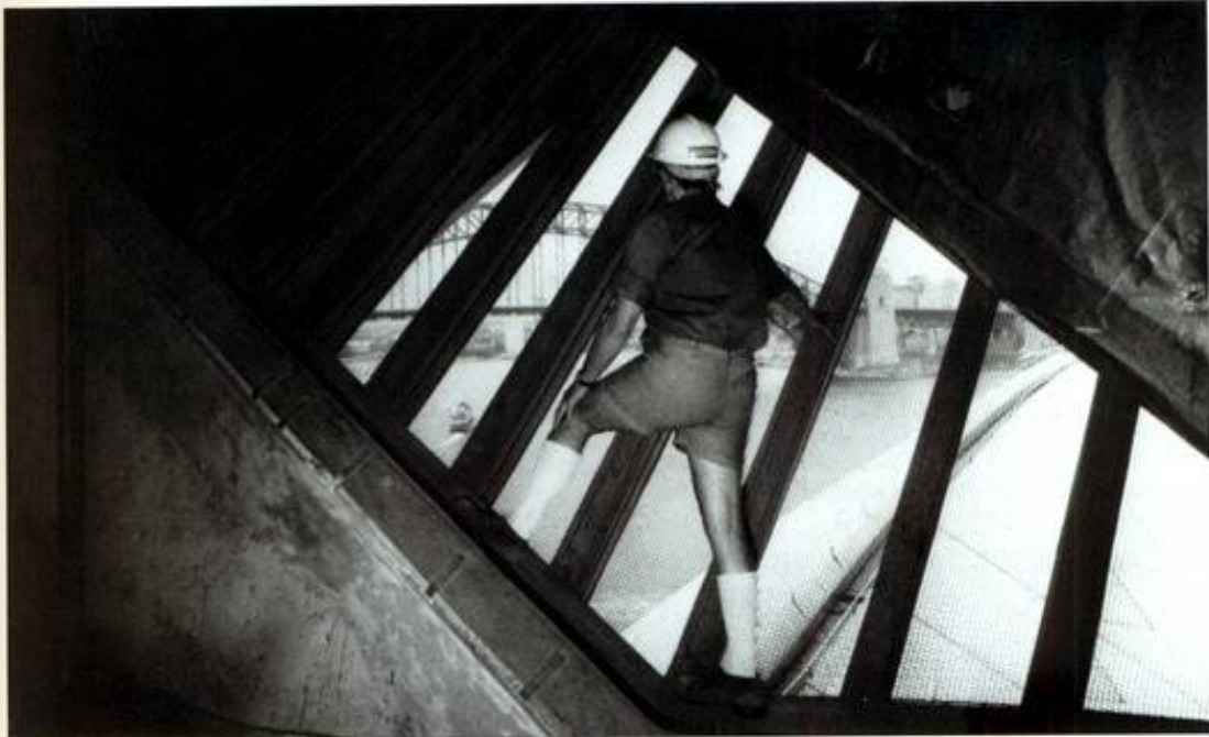
Main air intake, Sydney Opera House
