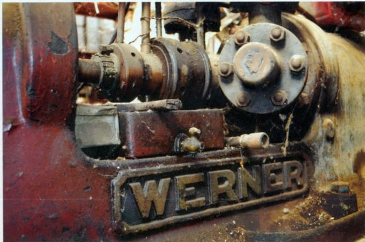
Werner Melbourne supplied two of three plant room engines.
