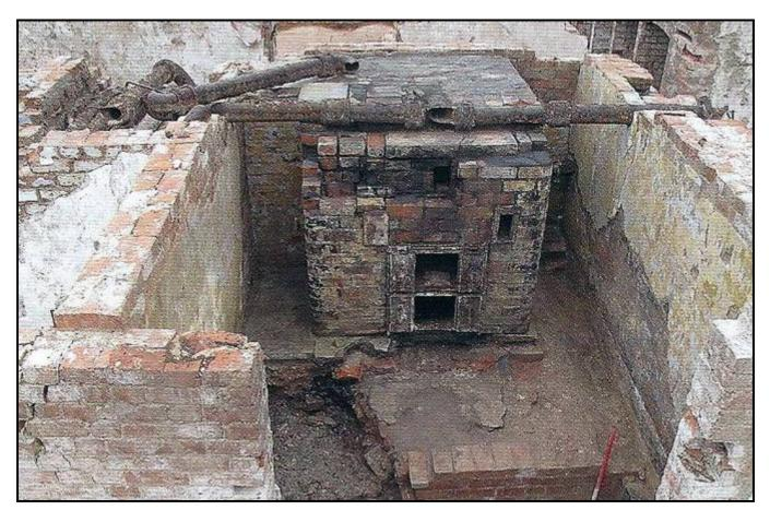
The basement at Worsley New Hall housed the hot water boiler, with heat exchanger coils in the chambers either side.
