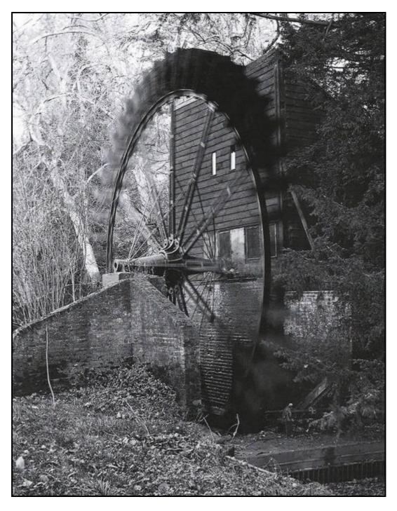
The cast-iron waterwheel, built by Bramah & Sons in the 1830s to replace the original horse-driven wheel which pumped water from the River Mole to the lakes at Painshill Park: (Photograph of 1899).
