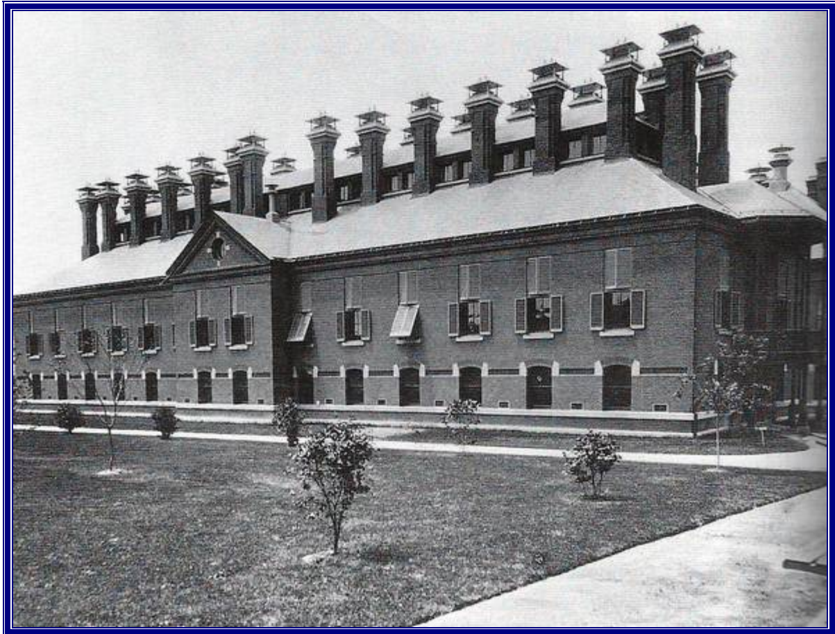
The prominent ventilation chimneys of Baltimore's John Hopkins Hospital
