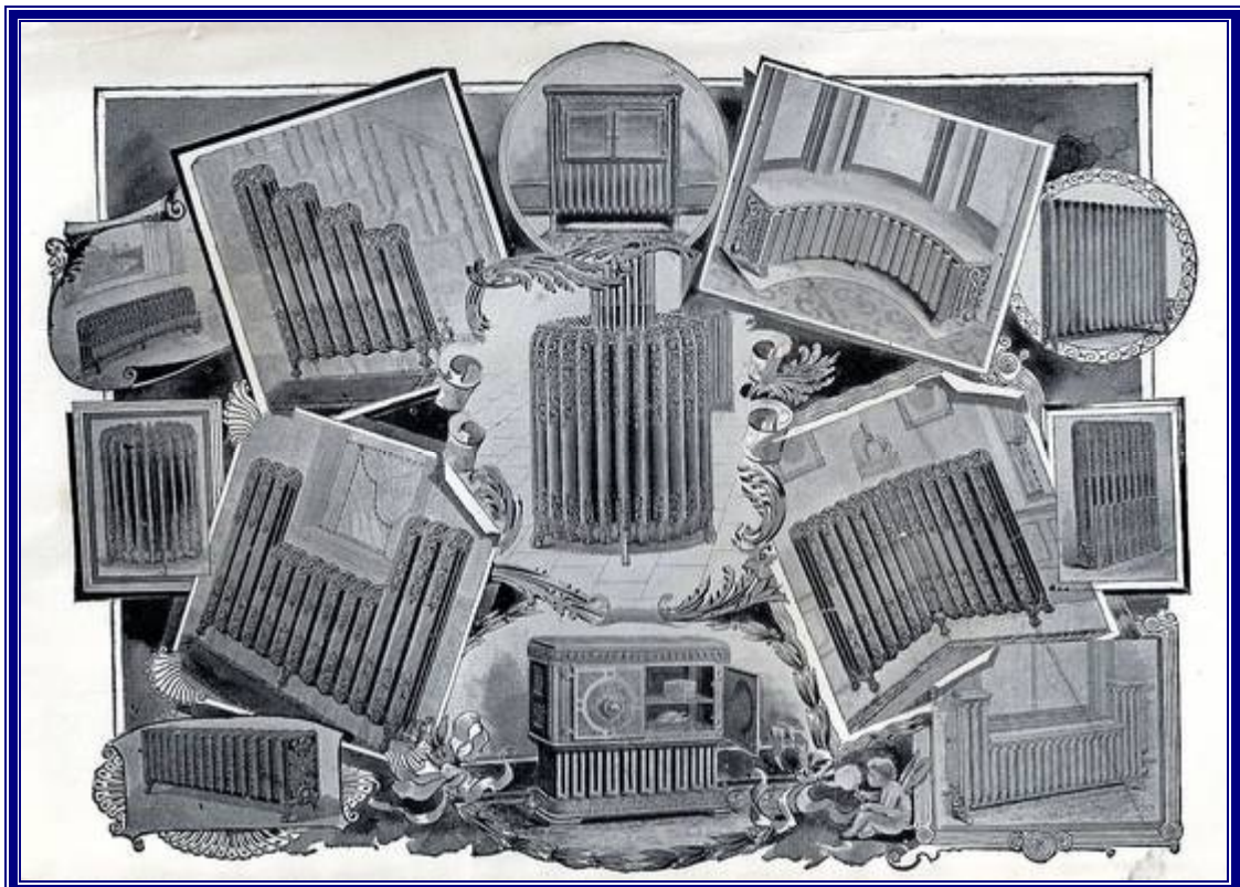
Cast-Iron radiators: frontispiece from the 1910 edition of Carpenter's H&V textbook
