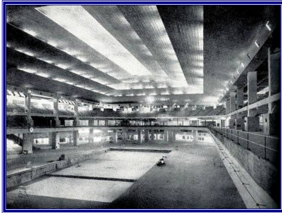
Earl's Court Main Hall with ventilation nozzles at high level
