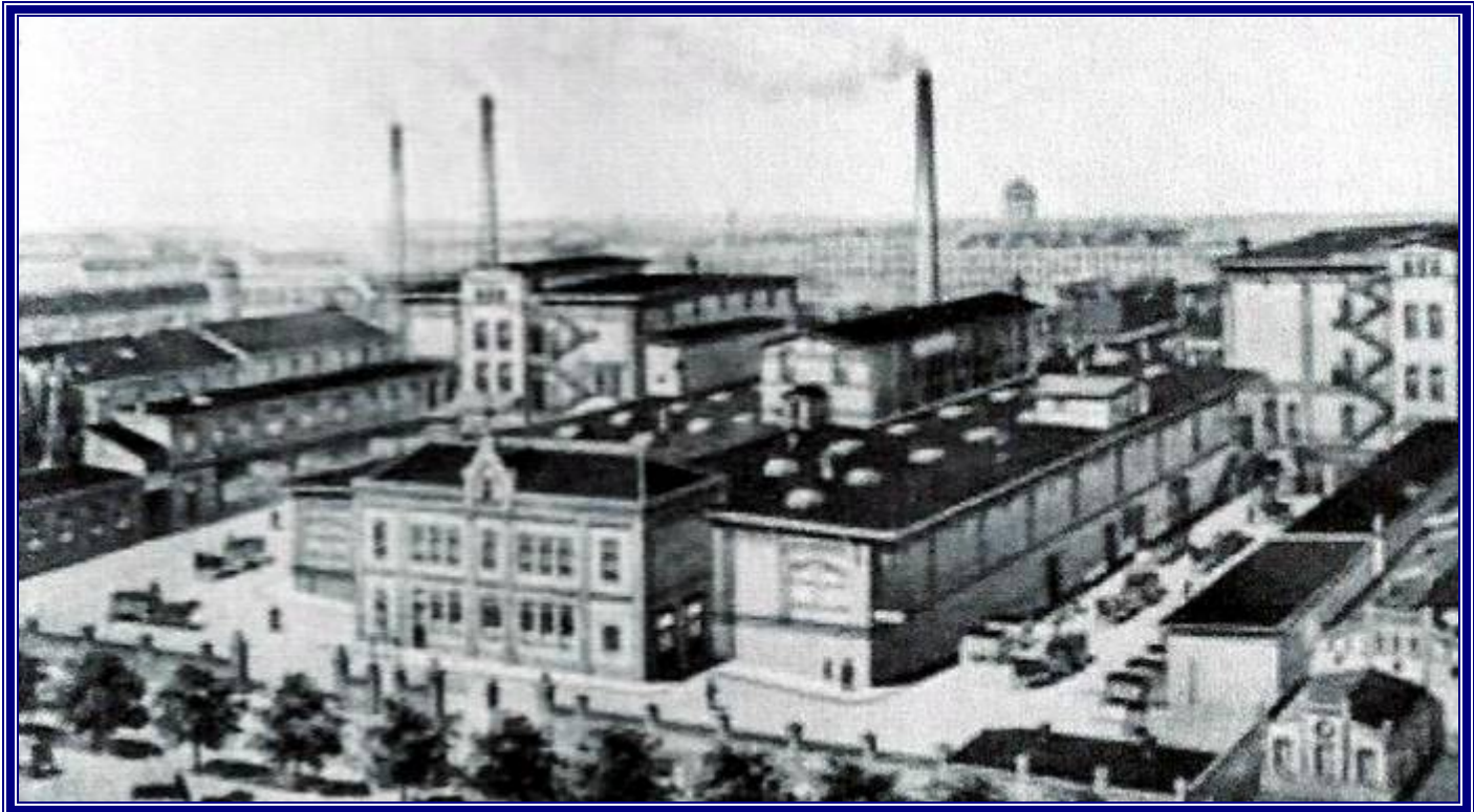
Linde Plant for Chilling Food & Ice-Making, Hamburg, 1892
