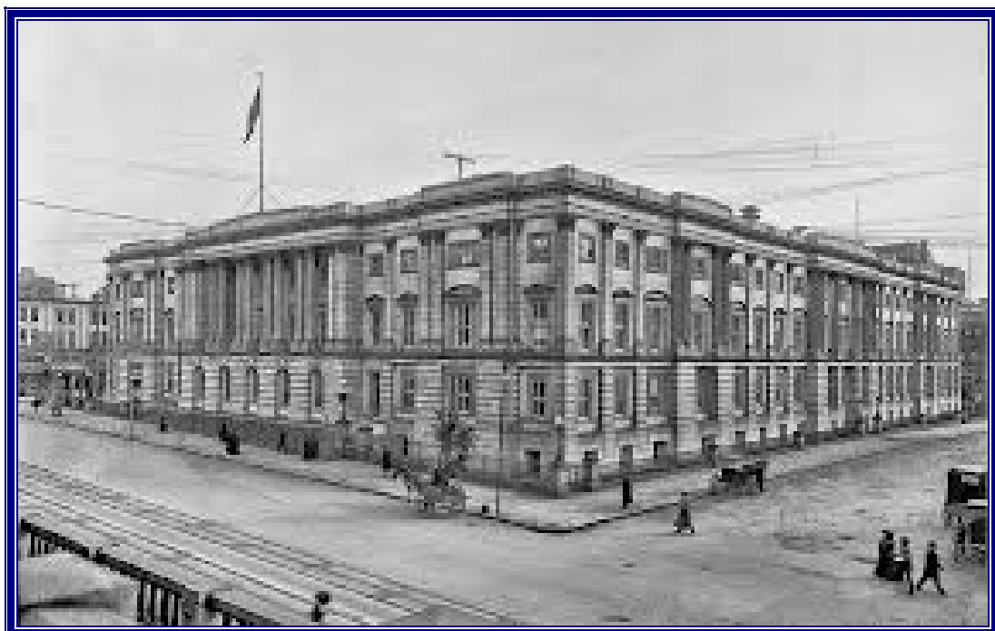
The General Post Office, Washington DC
