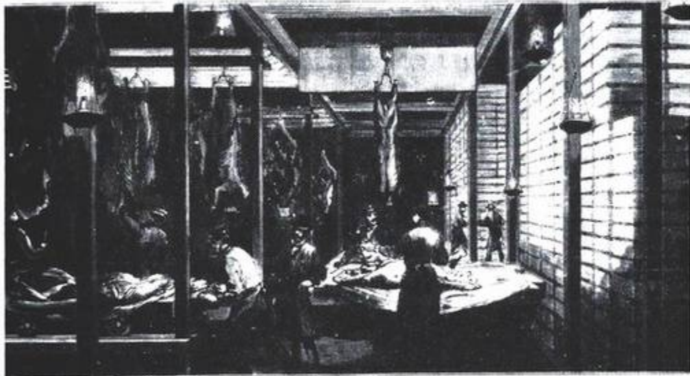
THE COLD AND FREEZING ROOM.
