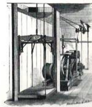
Metropolitan Hoisting Machine, showing Corner Platform. Cut K.
