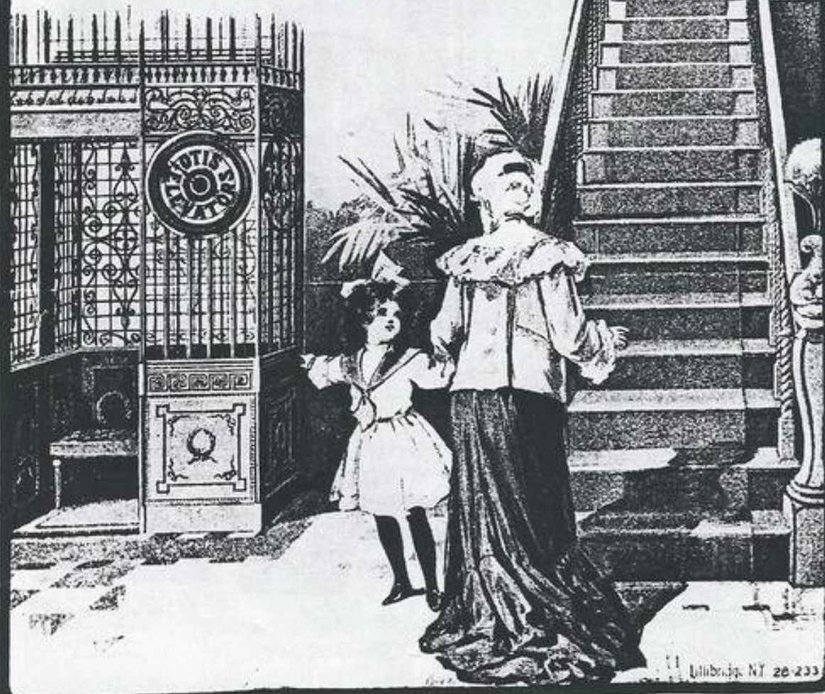
The Automatic Electric Elevator introduced in the 1890's
