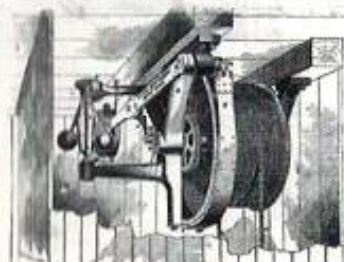
Automatic Safety Drum. Cut C. Old Patent Safety Platform for stores and high buildings where the excessive weight of the Wire Lifting Boys tends to prevent the Safety Spring from acting at the critical moment. Securely mounting a safety device immediately between the Hoisting Engine and Safety Platform necessary. This "Safety Drum" is secured directly onto the hookway and acts as a counter to the entire machine, instantly stopping the Platform upon any approach to its steady position.
