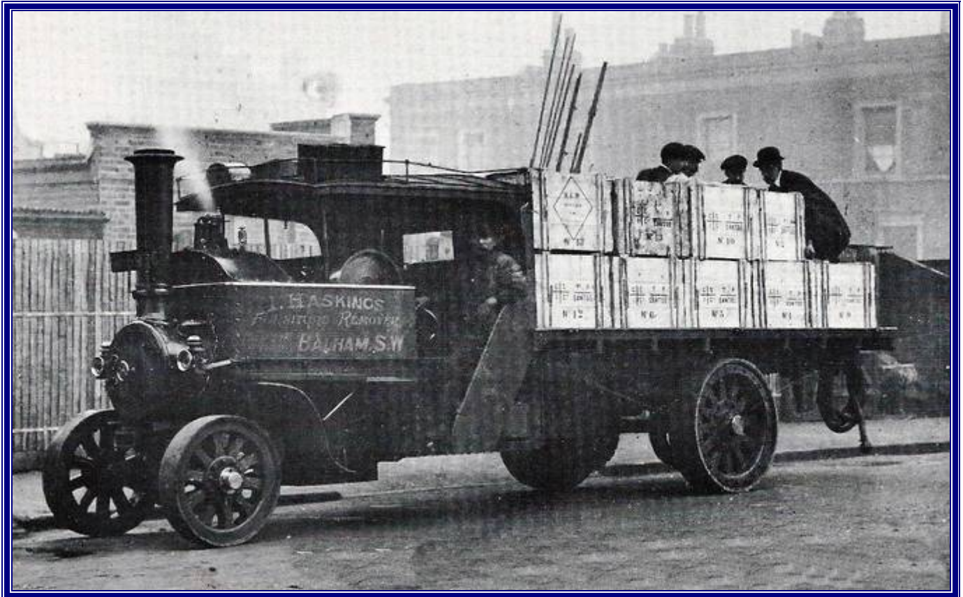
Delivering Potterton boilers in 1906
