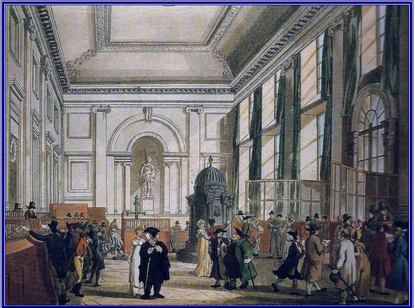
The Pay Hall of the Bank of England shown in a drawing by Thomas Rowlandson, published in 1808. In the background is a massive heating stove.
