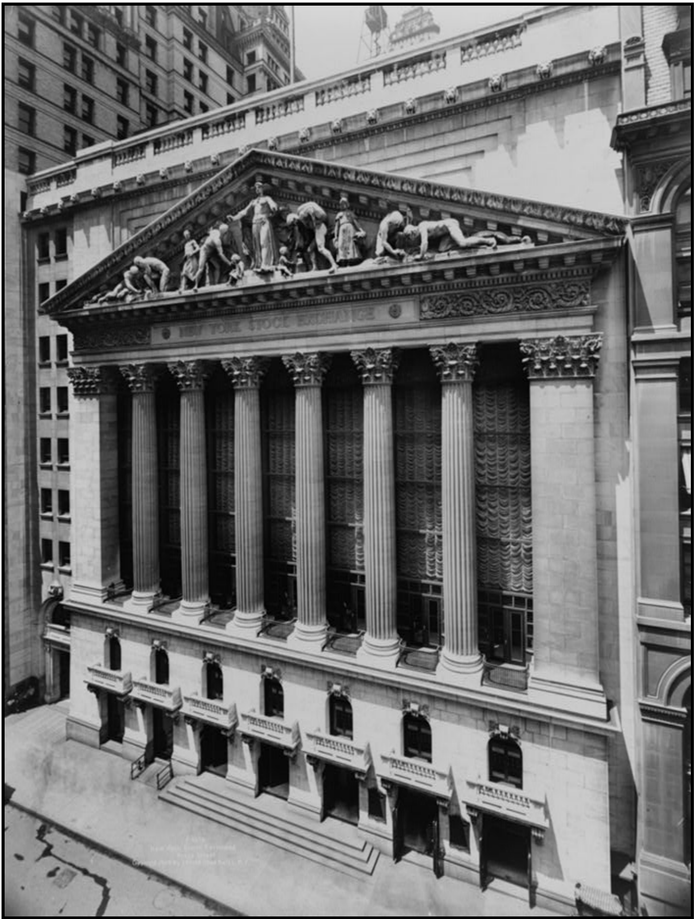
The New York Stock Exchange opened in 1903, with the first large-scale combined Air Conditioning & Co-generation system, designed by Alfred Wolff.
