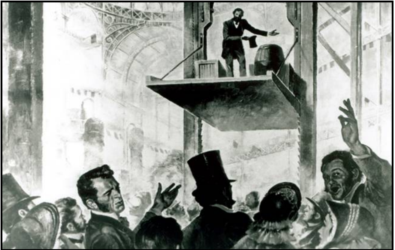
Otis demonstrating his safety lift "by cutting the rope" at the 1854 New York World's Fair
