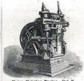
Union Hoisting Engine. Cut B. Old Patent Double-line Hoisting Engine, showing application of Patent Automatic Stop Mechanism, by which the engine is automatically stopped after making any desired number of revolutions. Motion of Platform of well of standard, up to 100 feet per minute.
