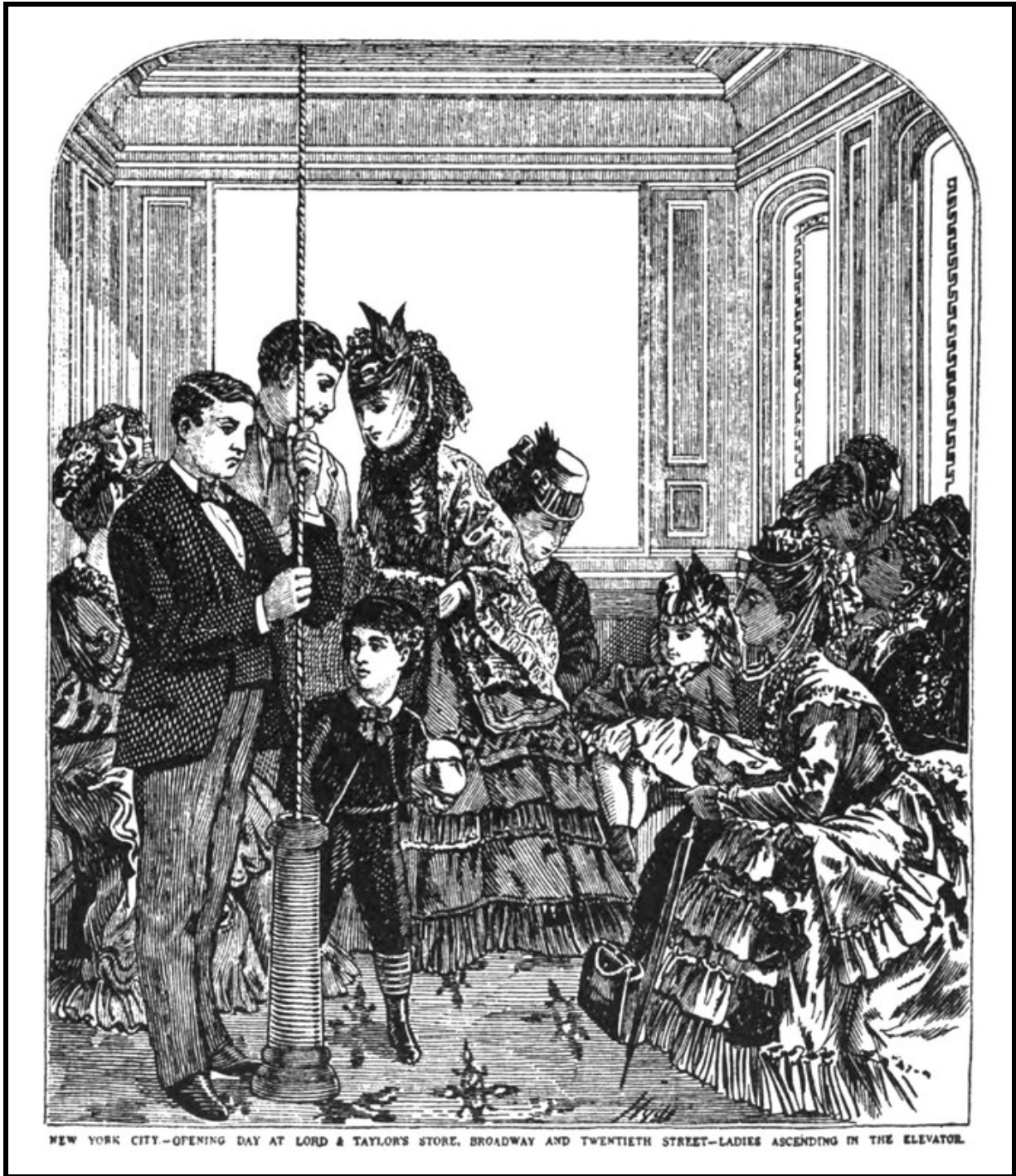
In 1873, Otis provided a steam-operated elevator with a manually controlled rope system for starting and stopping to serve the new Lord & Taylor Department Store in New York City
