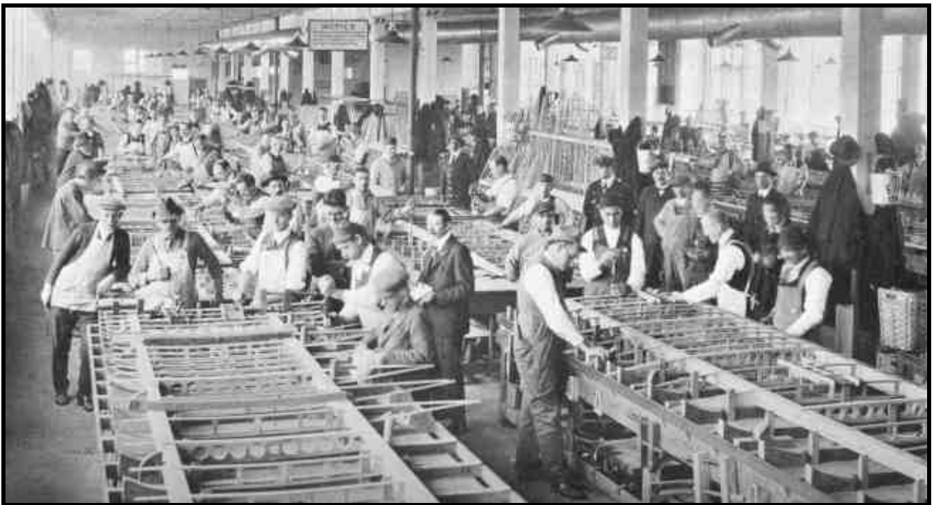
Sturtevant's Hyde Park Manufacturing Plant, early 1900's (Assembling aircraft wings in the lower photo)
