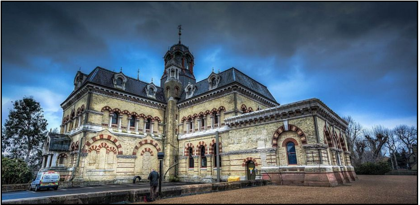
Abbey Mills pumping station (leepellingphotography)
