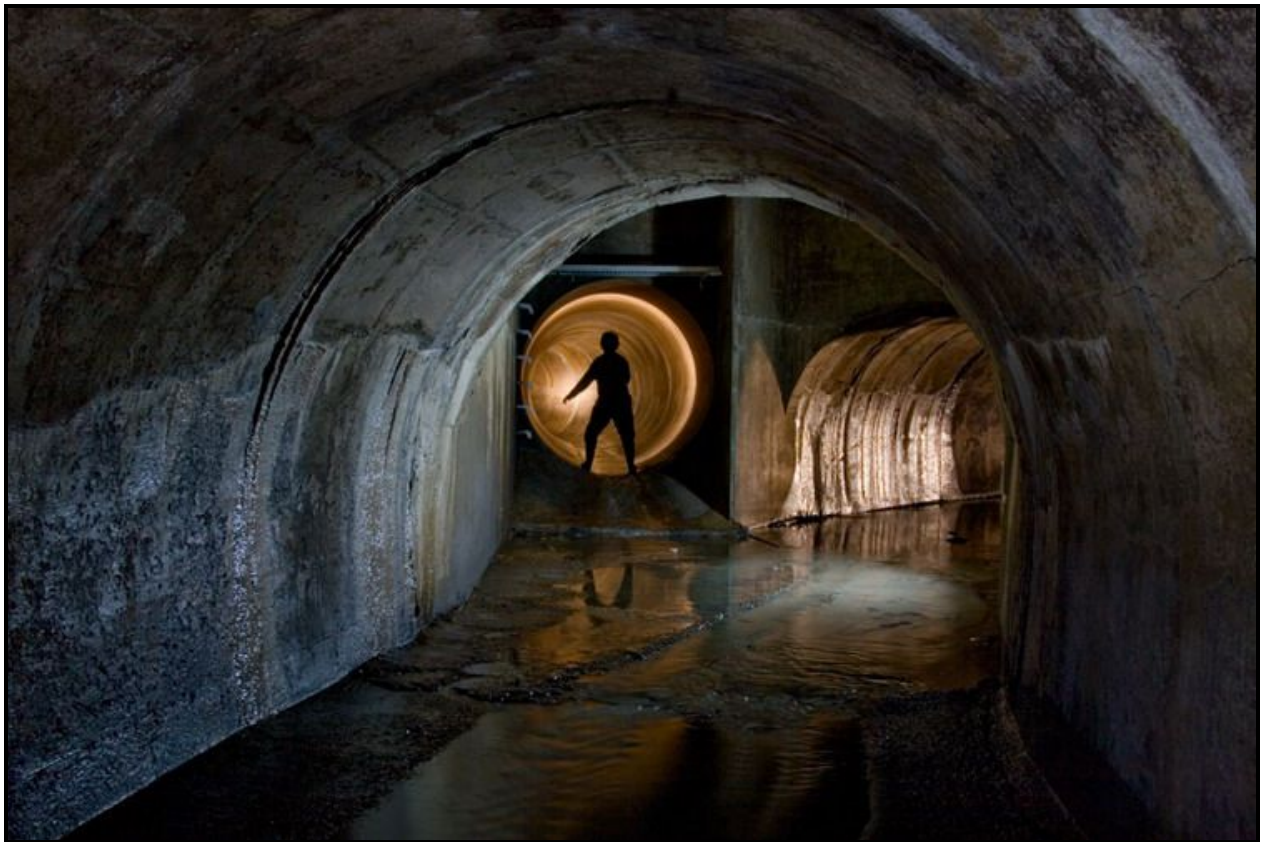
Modern photographs inside of London's main sewers
