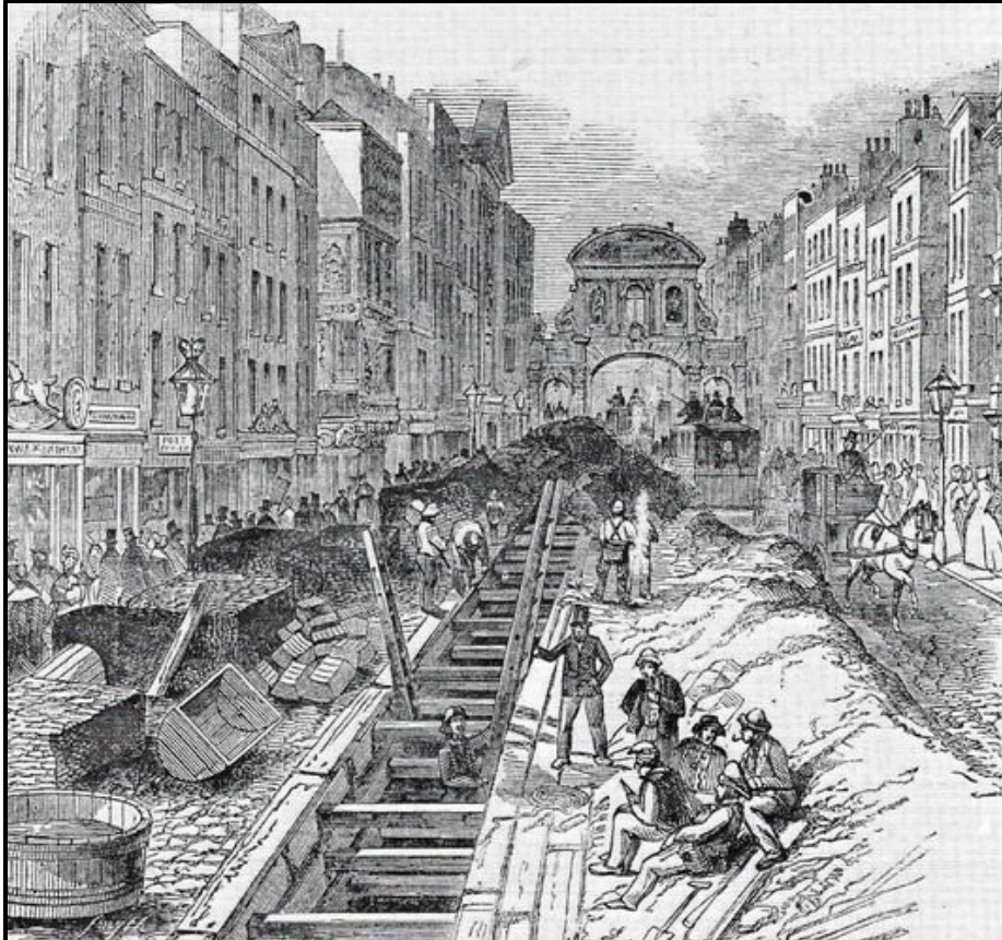
New sewers were constructed using the Cut and Cover method
