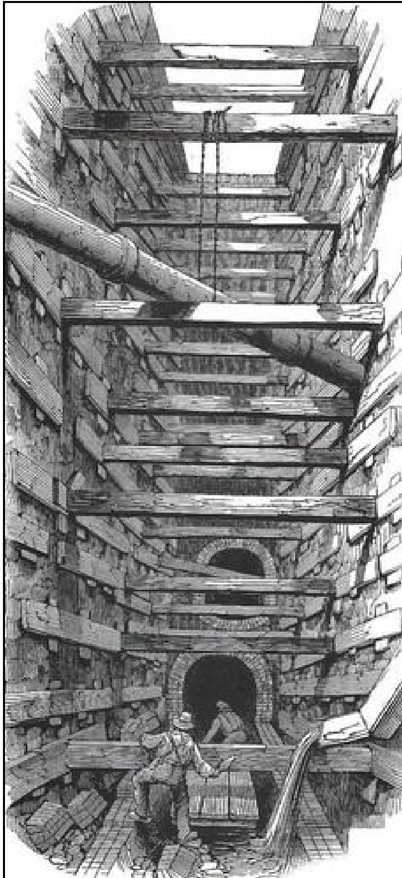
Sewers under construction
