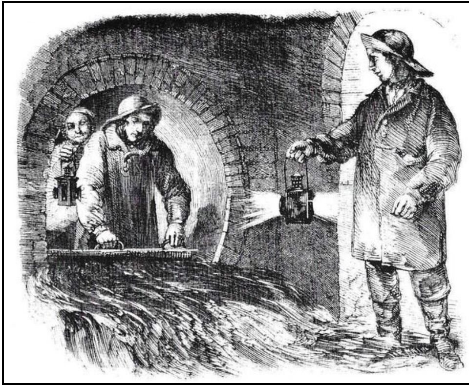
Existing sewers had to be flushed
