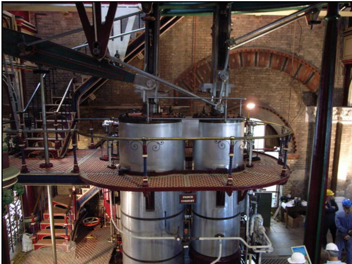
The Prince Consort pumping engine at Crossness
