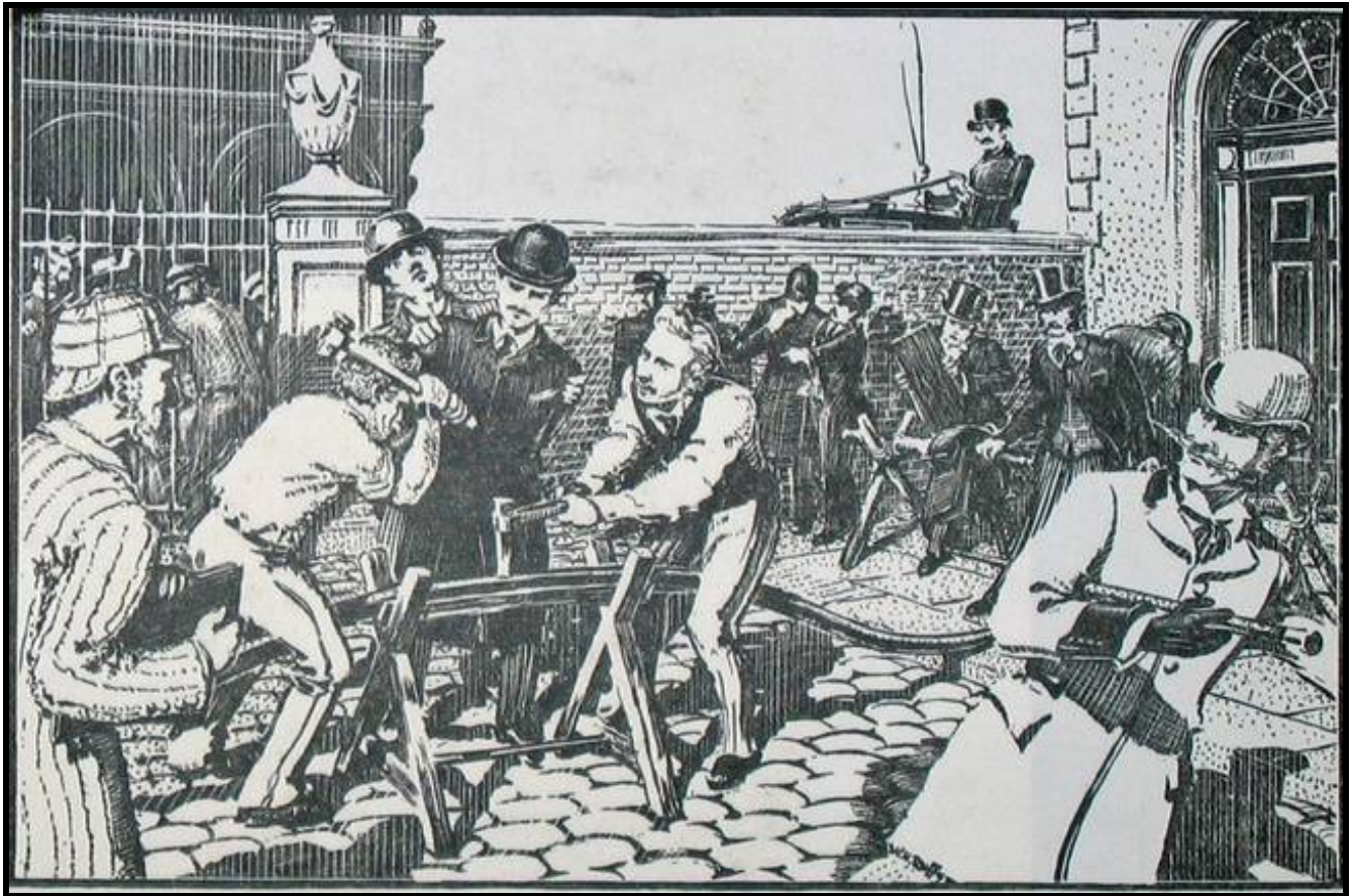
Demonstration to prove the safety of the Ferranti cable
