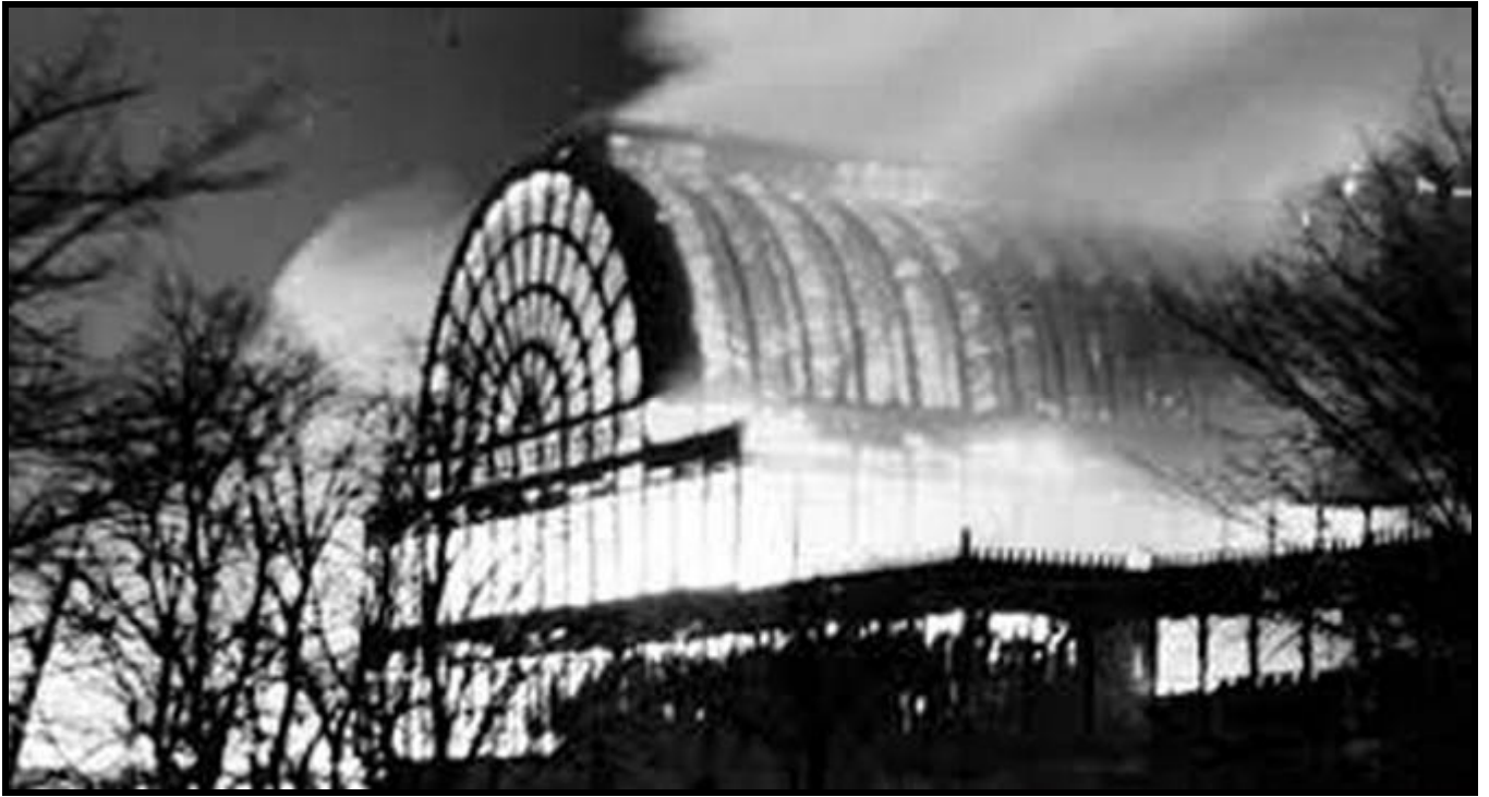
The fire raged out of control
