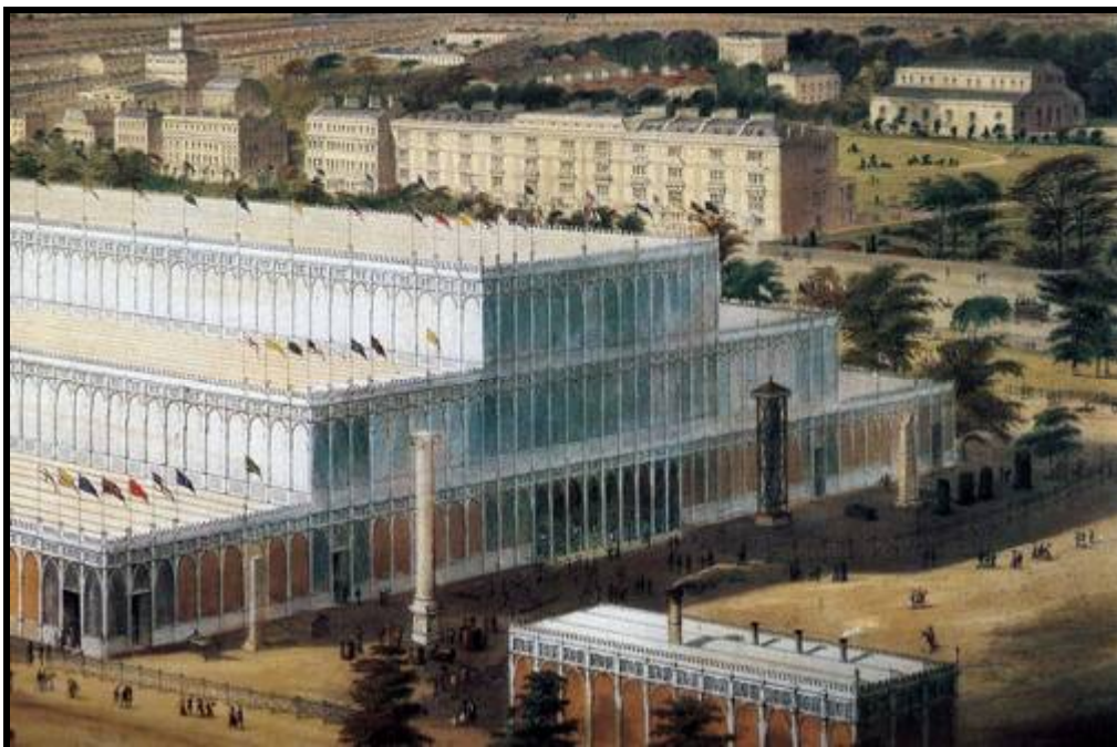
A corner of the Hyde Park Crystal Palace with its external boiler house
