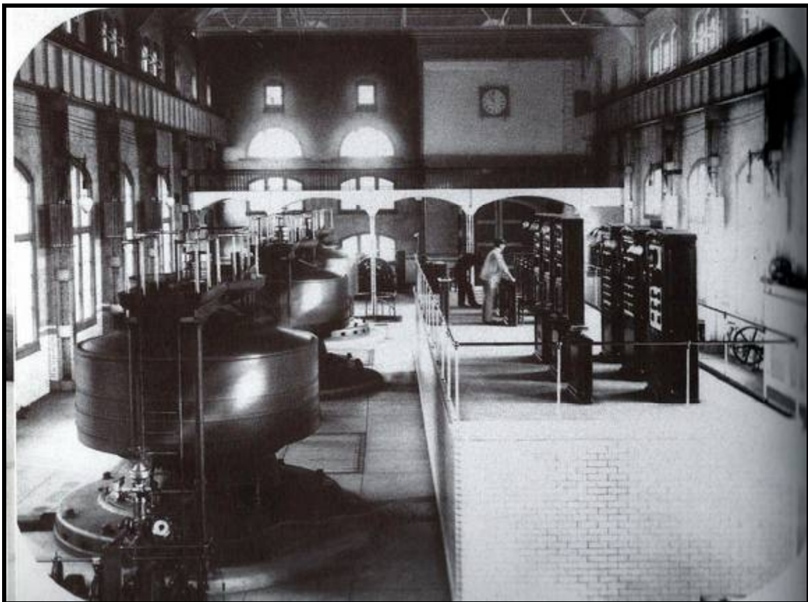
The first three Niagara Falls generators went on line on 16 th November, 1896
