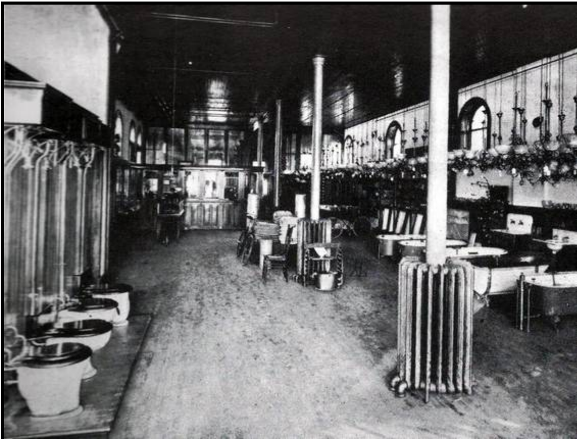
The Trane Plumbing & Heating Store
