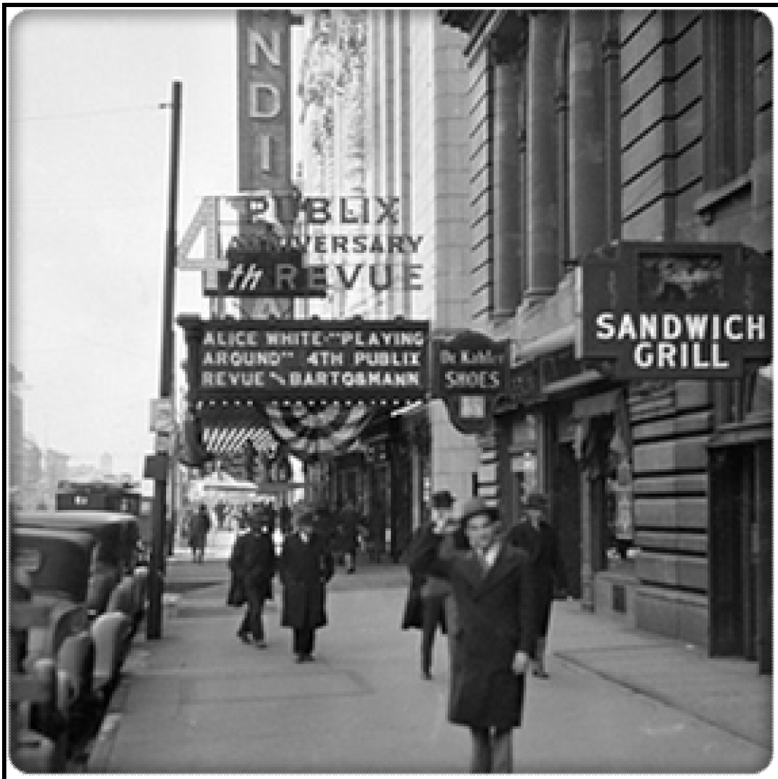
In 1931, Trane provided a "Cooling Coil System" for the Indianapolis Theatre
