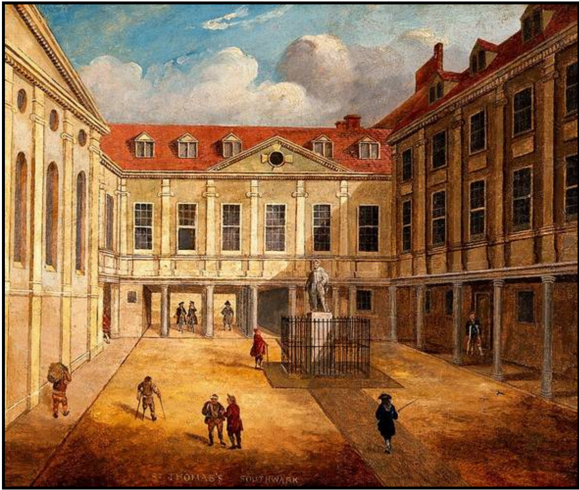
The original St Thomas's Hospital in Southwark, 1225-1865
