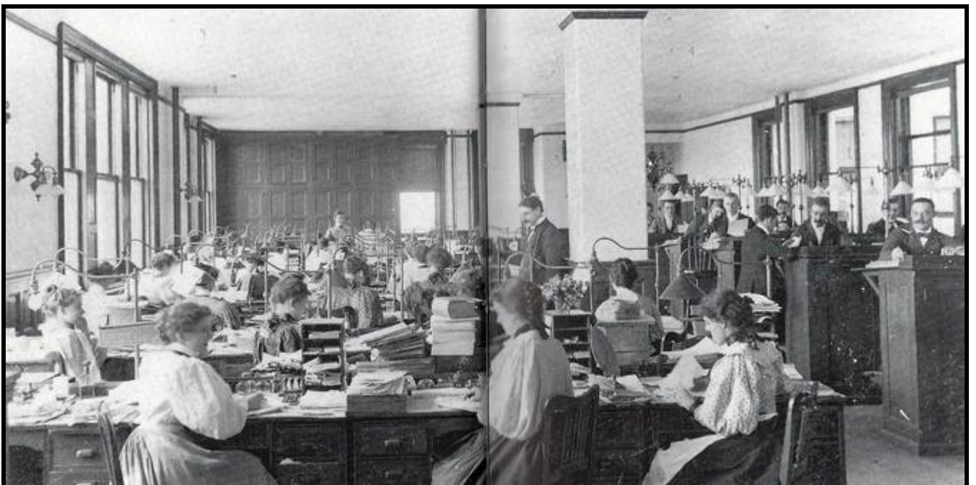
Workers in the former Metropolitan Life Insurance Building in 1896 (note lamps at each station) Replaced by the New Building & Tower of 1909 on the same site
