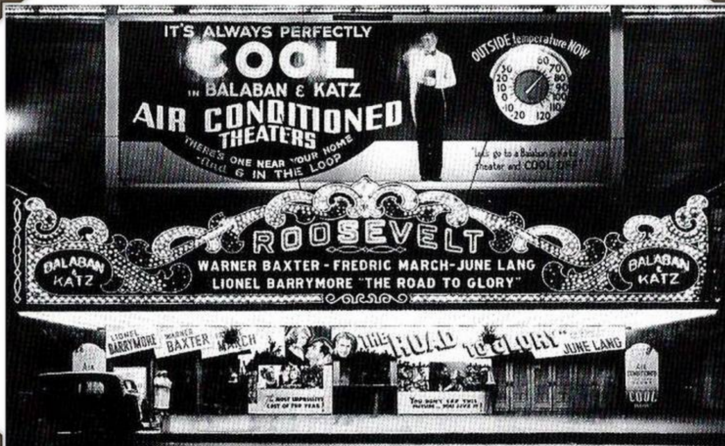
Comfort air conditioning, the Balaban & Katz "Roosevelt," Movie Theatre, Chicago, 1936
