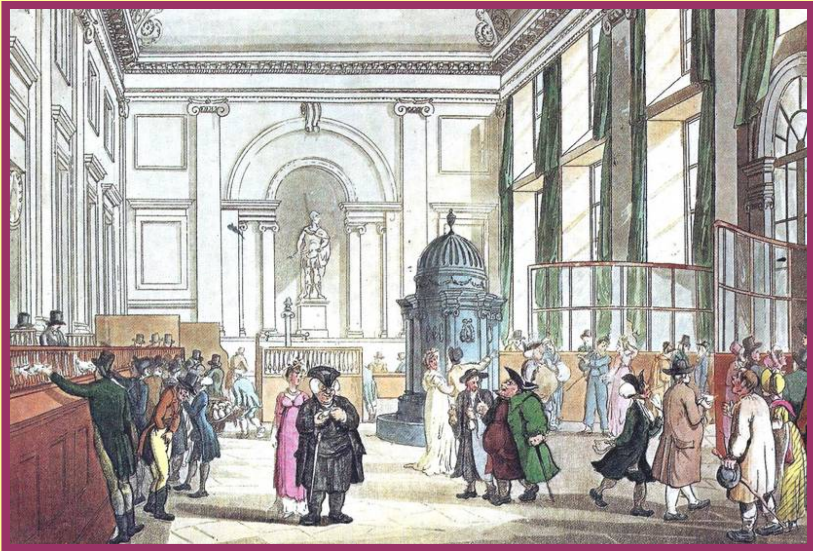
The Pay Hall at the Bank of England in London, complete with a gigantic heating stove, 1808
