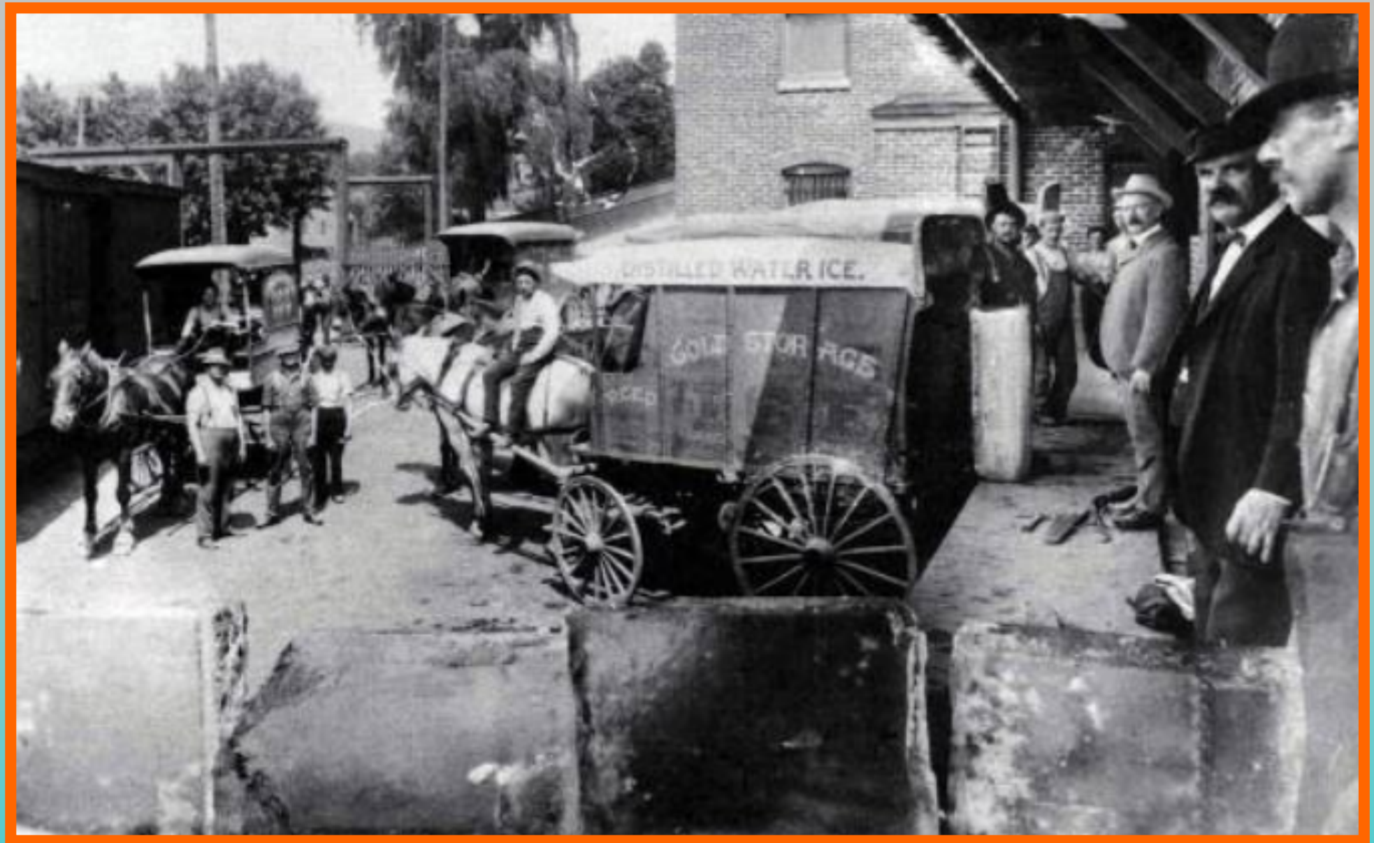
Loading ice at the Keystone Cold Storage Company, Reading, Pennsylvania, 1900
