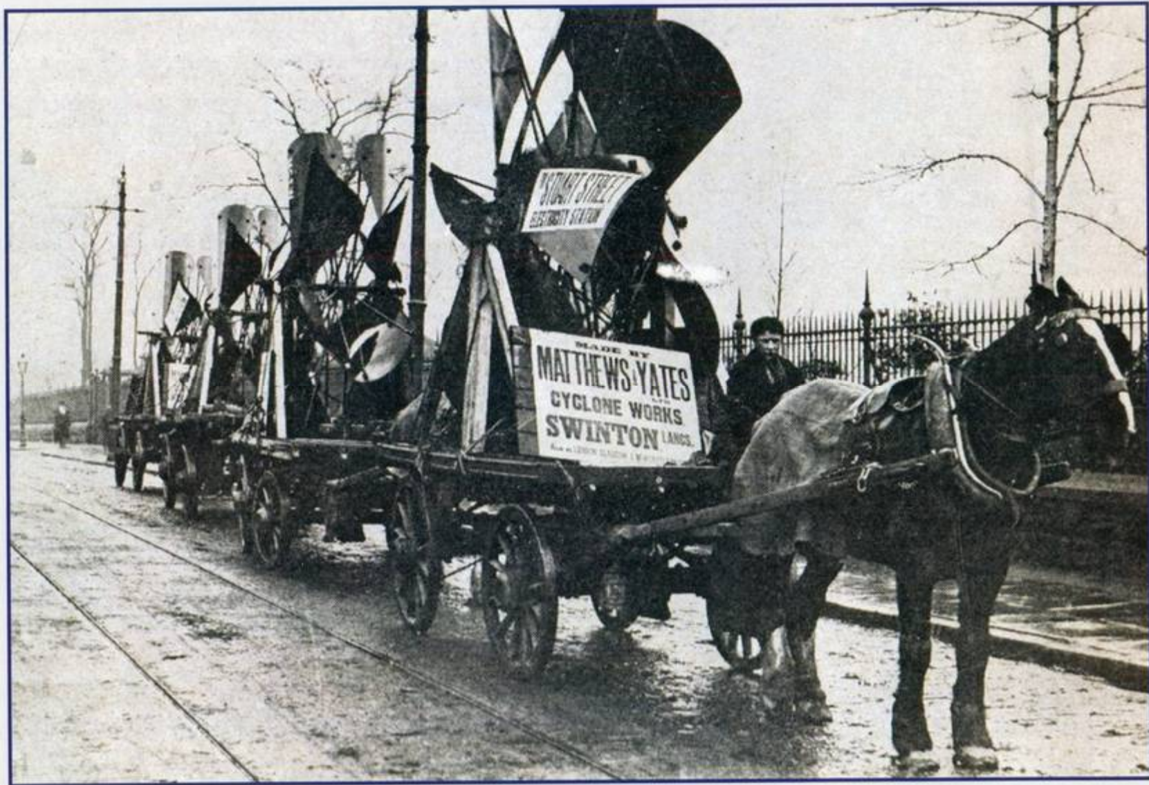
Delivering fans to an Electricity Station, Manchester, about 1895
