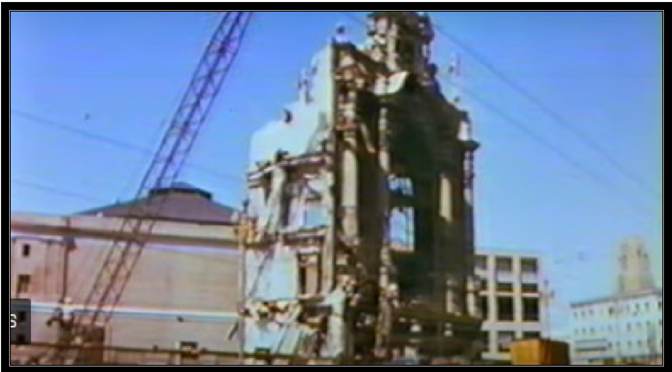
Demolition (video capture from YouTube; The Fabulous Fox)
