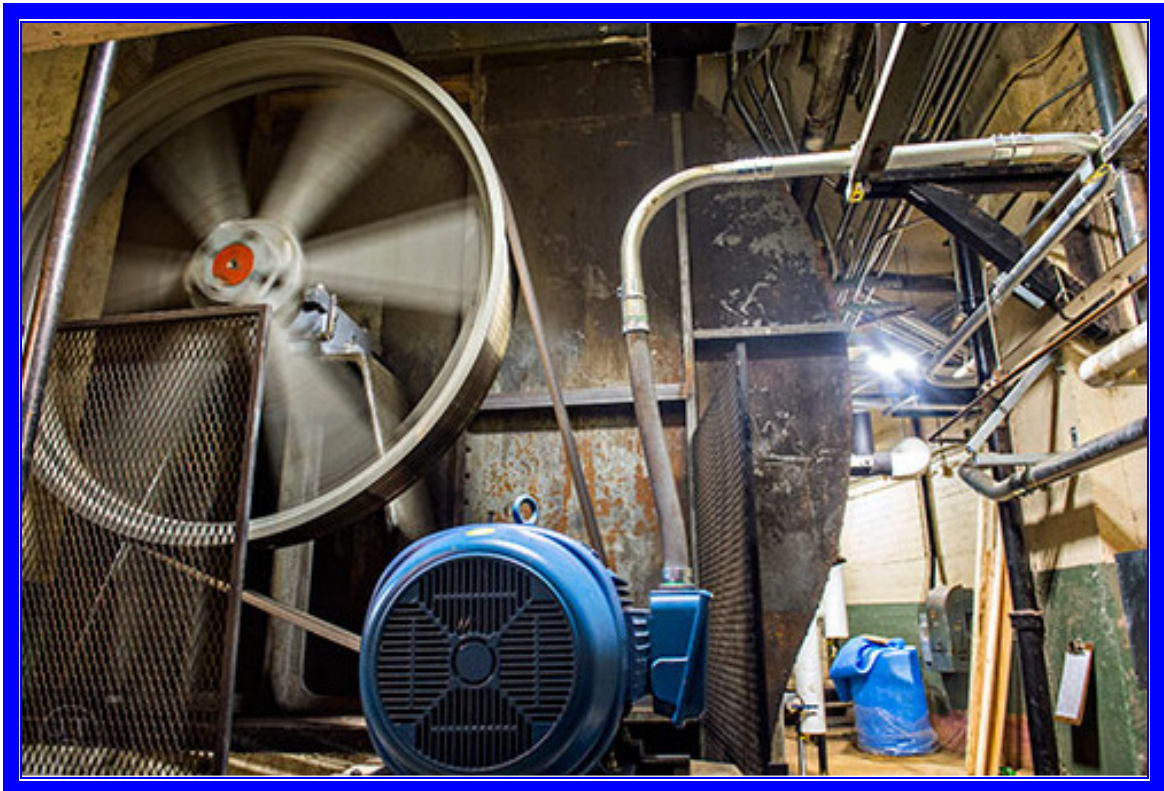
"A giant flywheel is now used to produce the energy for the air conditioning" ? (Text on website)
