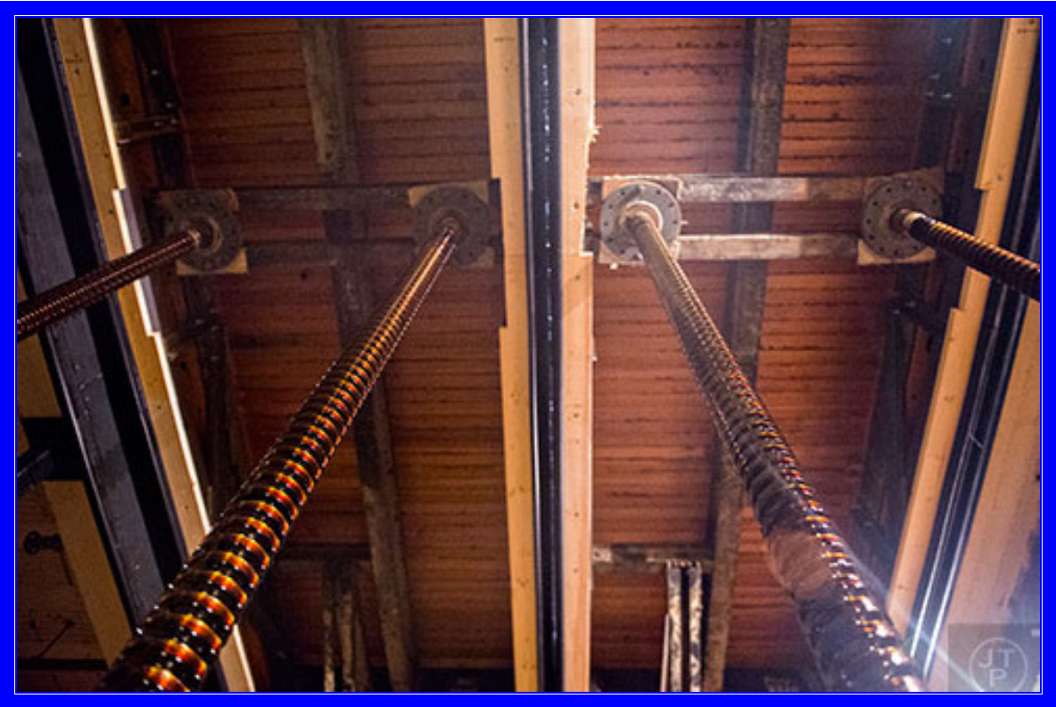
The screw-type stage lifting mechanism
