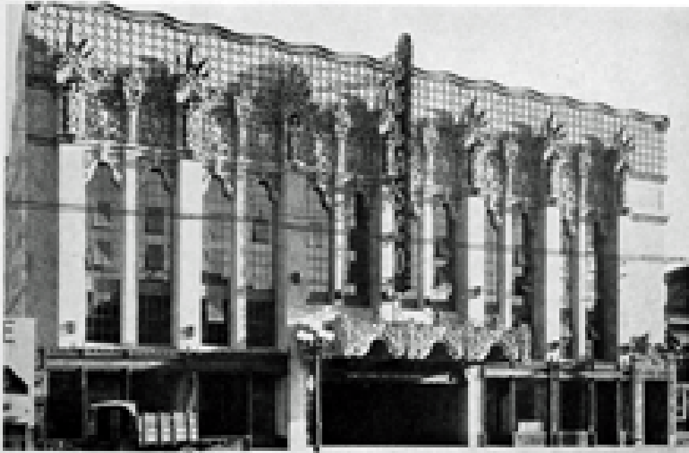
BELASCO THEATRE, ONE JOHNSON Mason, Walls and Floors, Scaffolding
