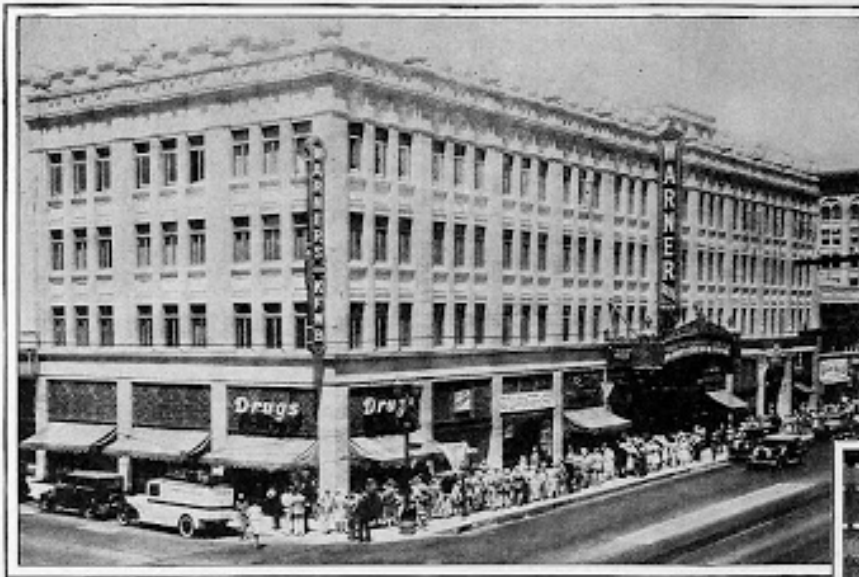
Warner Bros. Theatre, Hollywood, Calif., one of the most impressive theaters in the world, is equipped with C-H Dimmers. G. Albert Lamborgh of Los Angeles was the architect, English Electric Company, also of Los Angeles, were the contractors.
