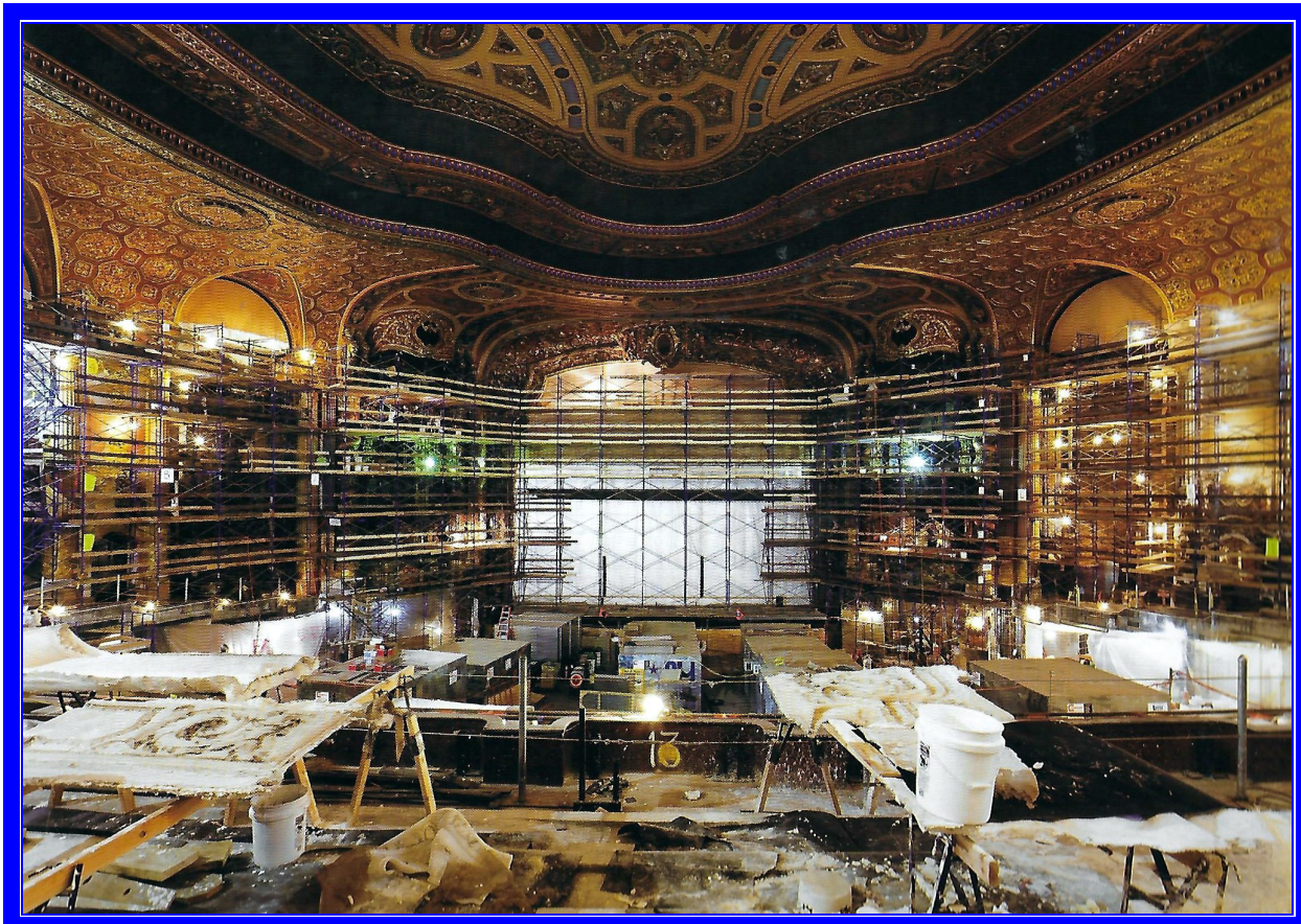
The auditorium with restoration in progress (KTML)
