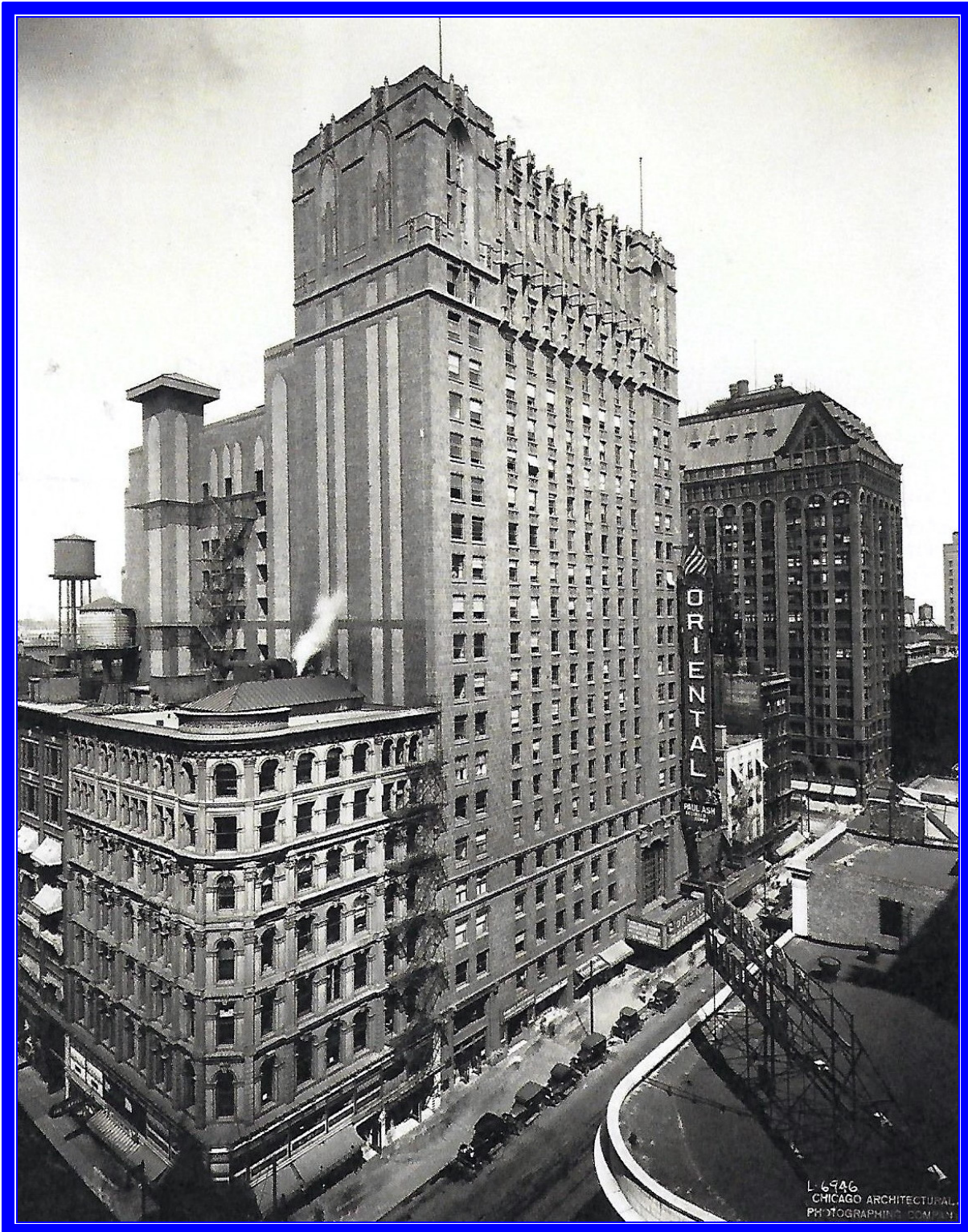
An example of a Rapp & Rapp design is Chicago's Oriental Theatre & Masonic Building, 1926
