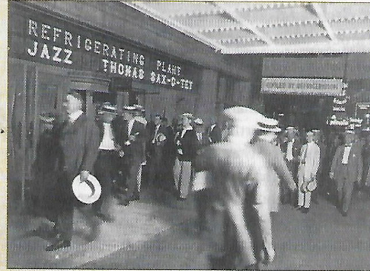
Figure 2 Rivoli Theater. The theater's refrigeration plant was prominently featured on opening day on Memorial Day in 1925. Source: Cool: How Air-Conditioning Changed Everything [Carrier]
