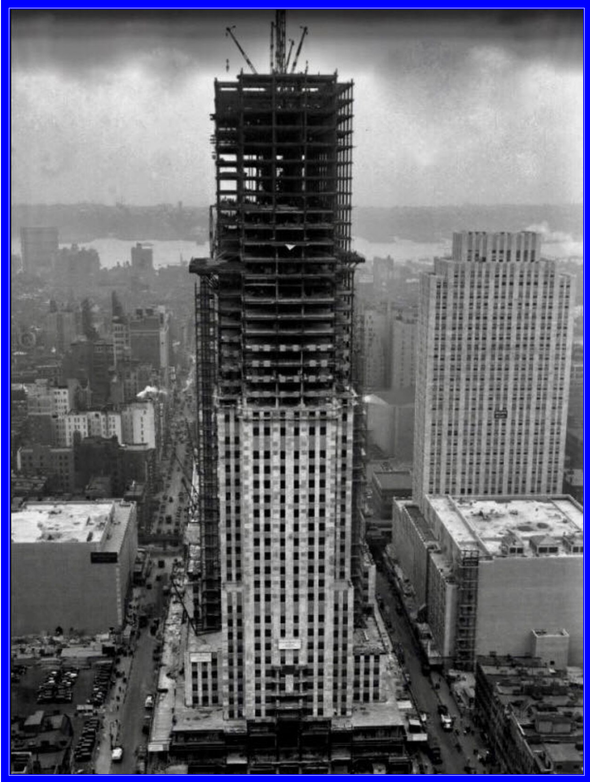
Building the RCA Tower
