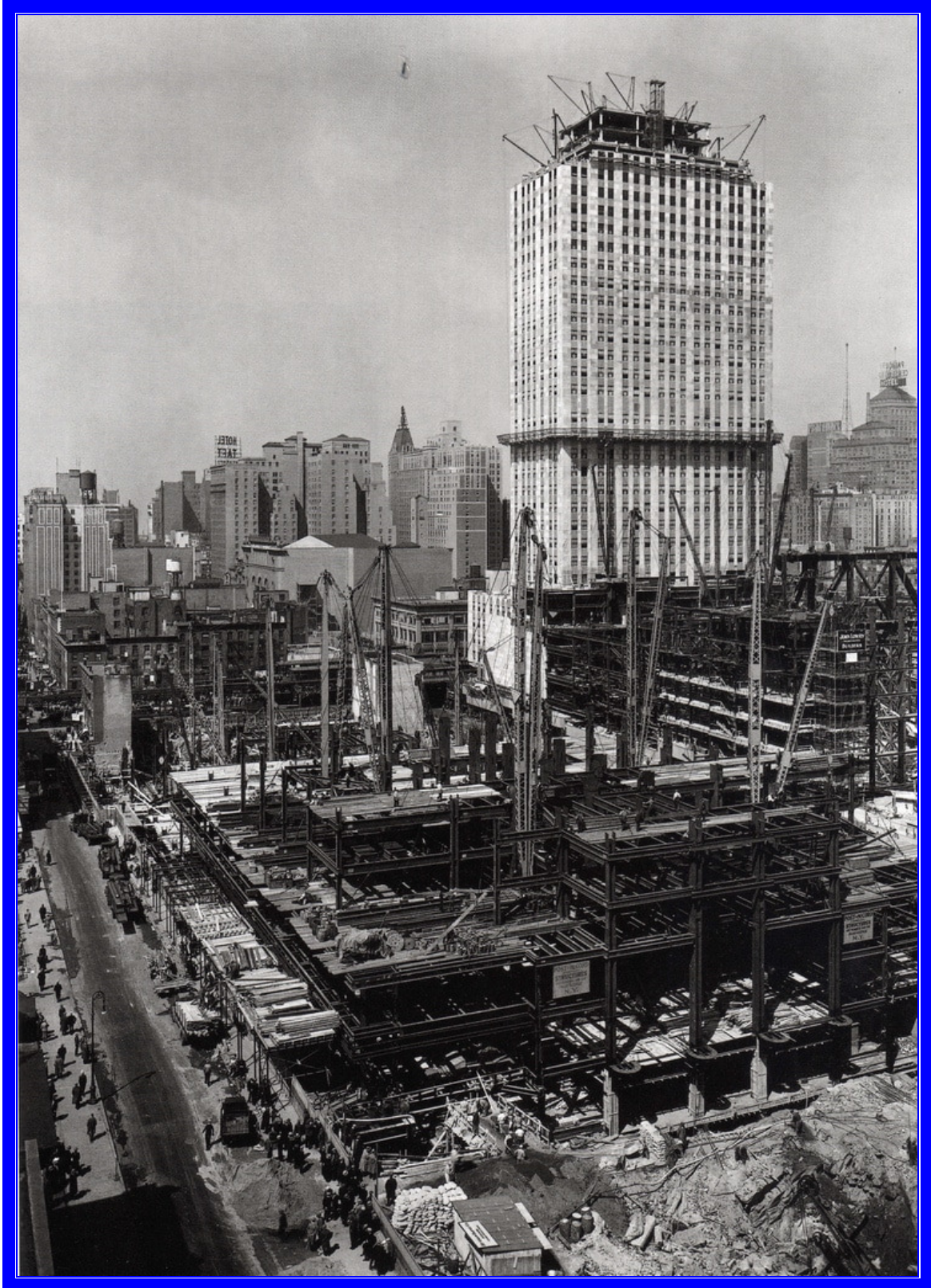
The 66 storey RCA Tower around the halfway stage
