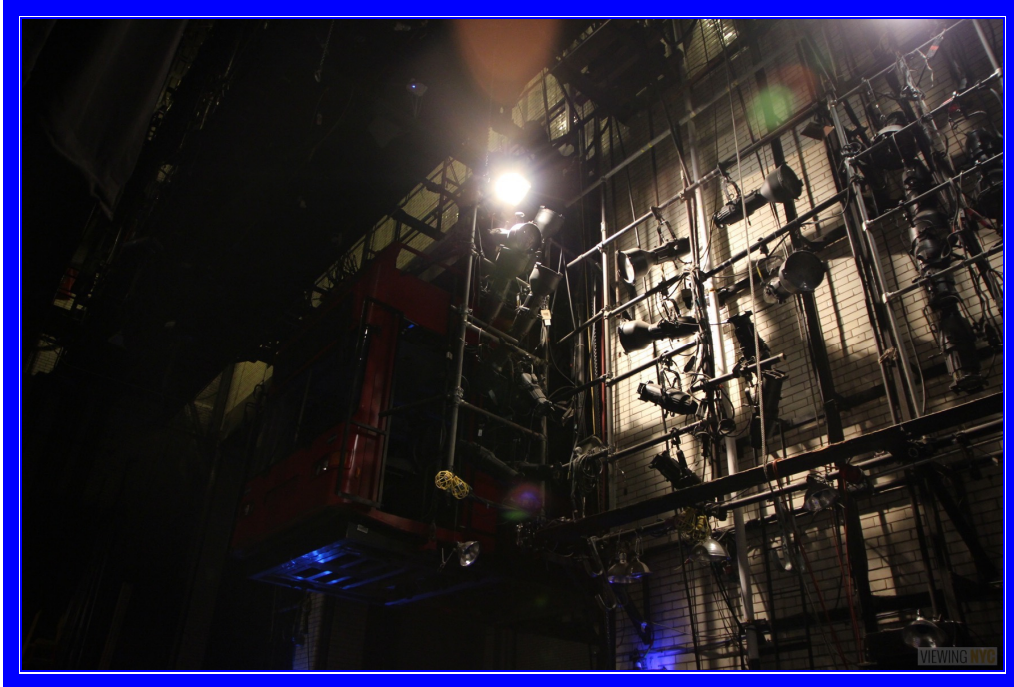
Stage lighting rig
