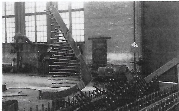
PIPE SECTIONS READY FOR INSTALLATION ON THEATRE RINK
