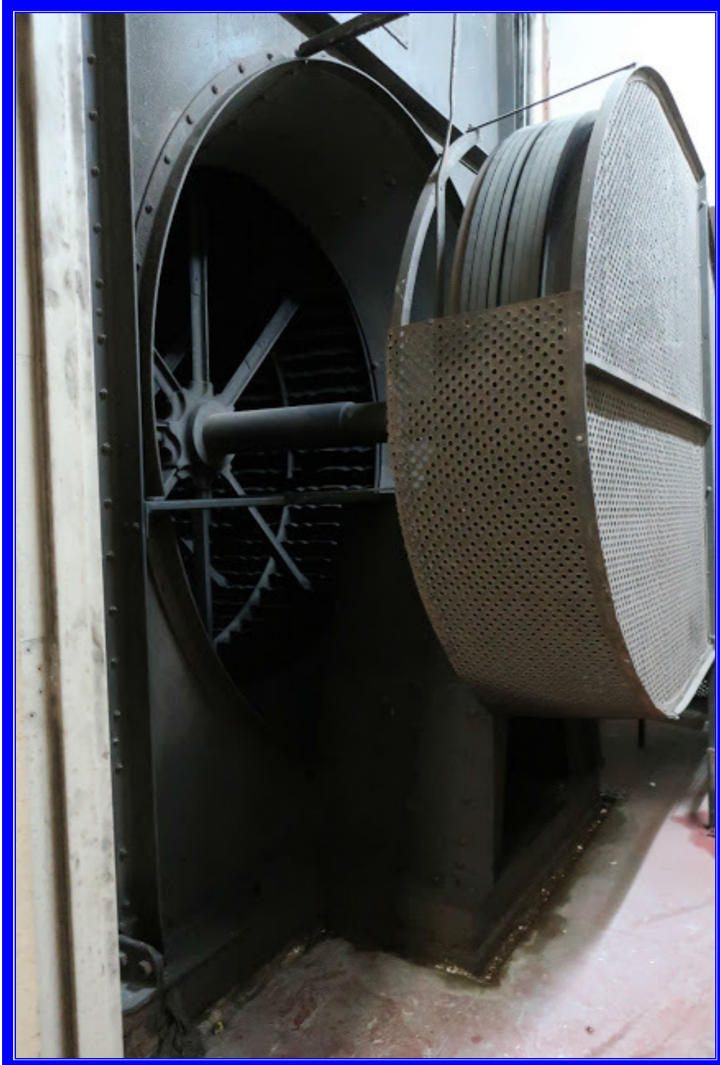
Centrifugal fan and drive guard
