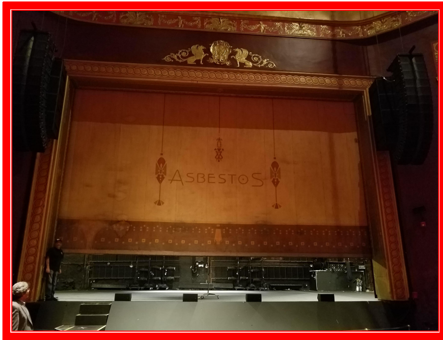
Asbestos safety fire curtain in old theatre installed to prevent or delay a stage fire entering the auditorium giving the audience time to exit the theatre in safety
