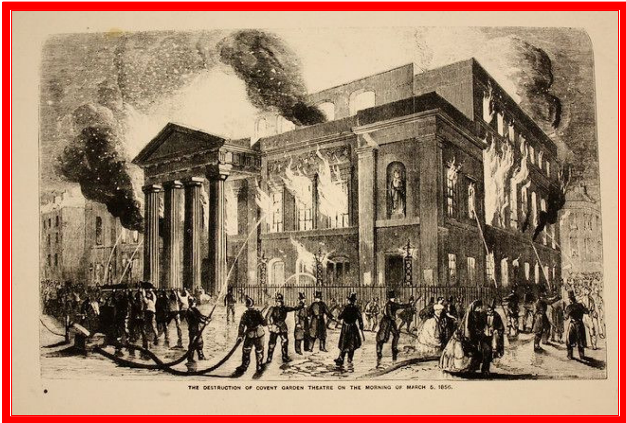
Covent Garden Theatre, London 1809, on fire 1856
