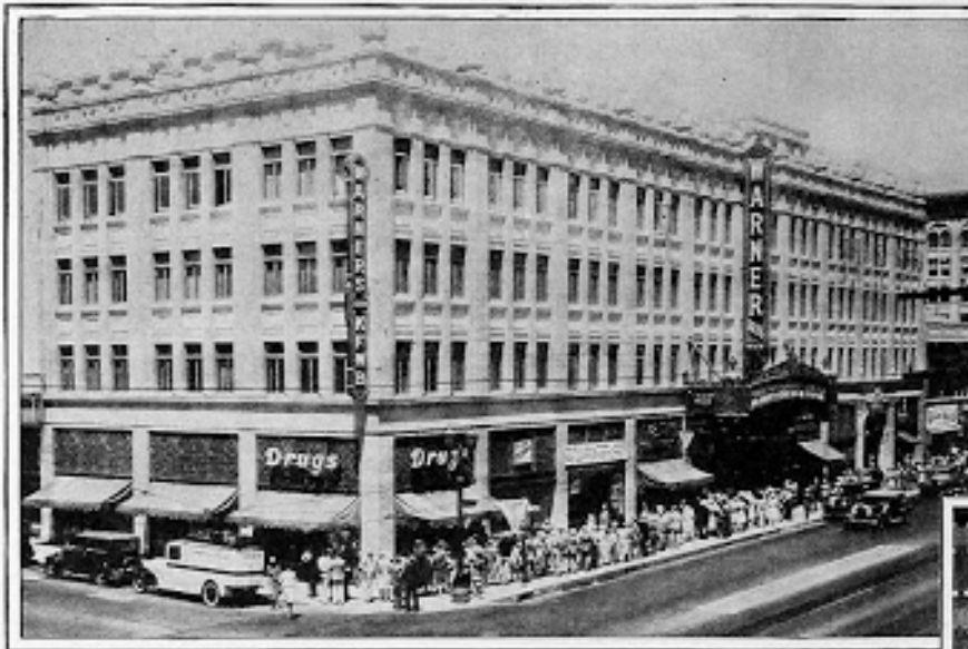
Warner Bros. Theater, Hollywood, Calif., one of the most impressive theaters on the West Coast, is equipped with C-H Dimmers. G. Albert Lamborgh of Los Angeles was the architect, English Electric Company, also of Los Angeles, were the contractors.
