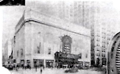
The Stanley, Pittsburgh, built by Hoffman-Hansen Company for the Stanley-Dauer-Clark Corporation. Complete York air cooling and air conditioning equipment installed.
