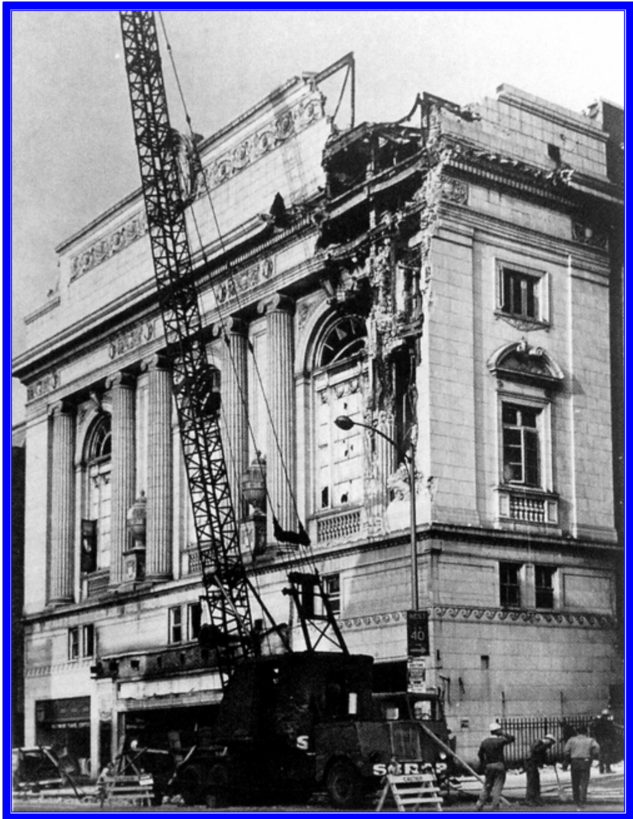
The start of demolition
