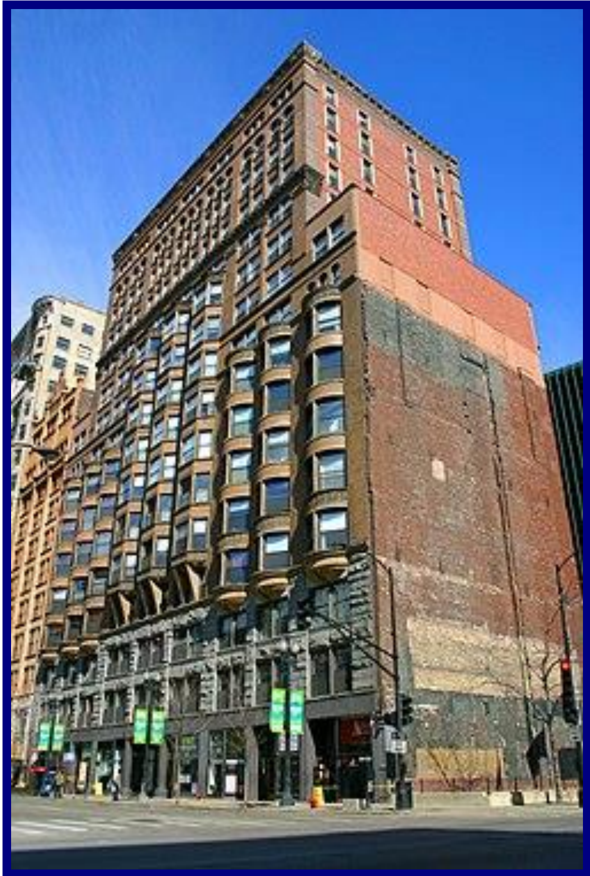
16 floors. Architect: William Le Baron Jenney. Oldest skyscraper with "purely skeletal structural system."
