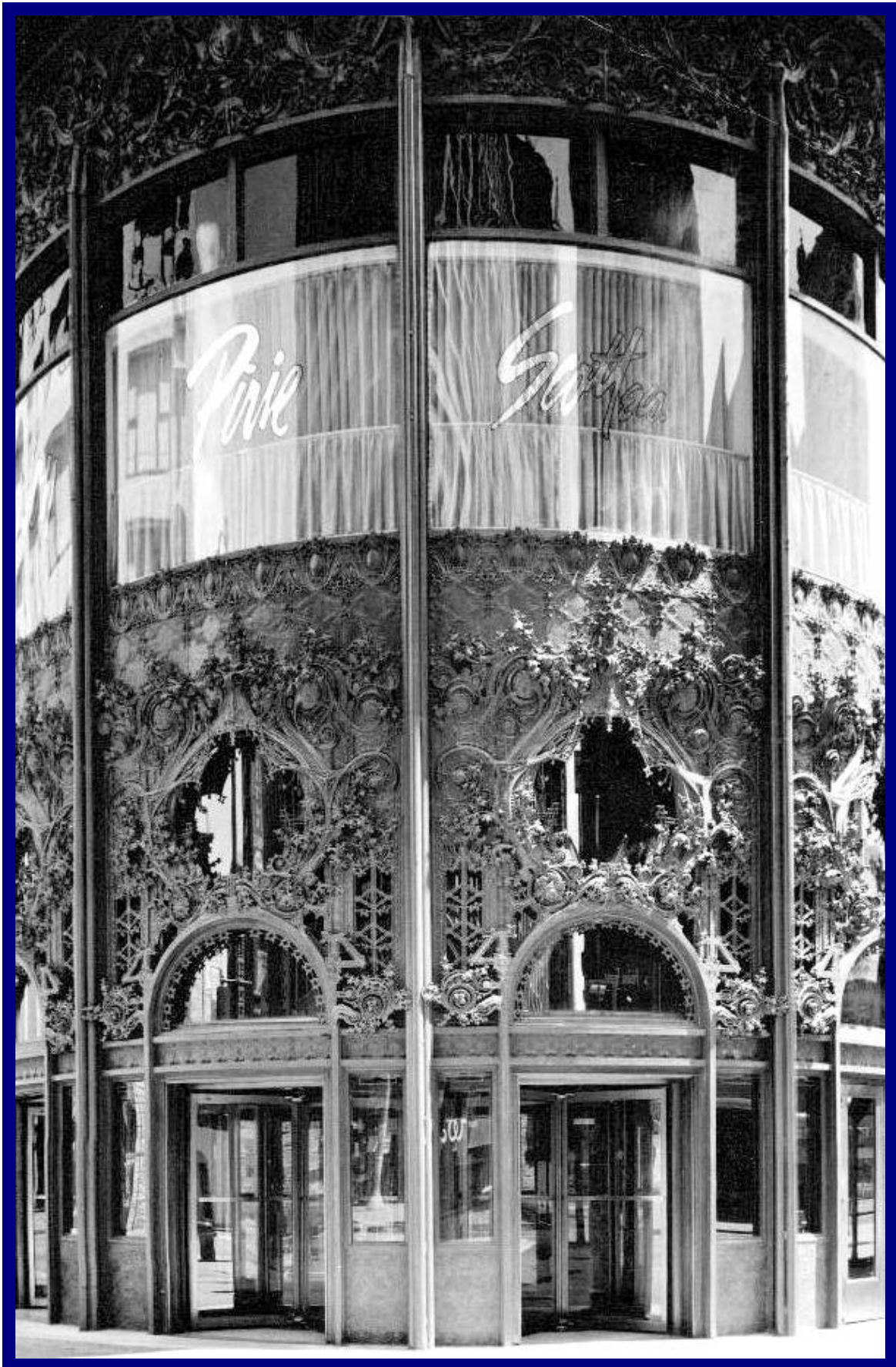
Architect: Louis Sullivan. Building included a very early fire suppression sprinkler system.
