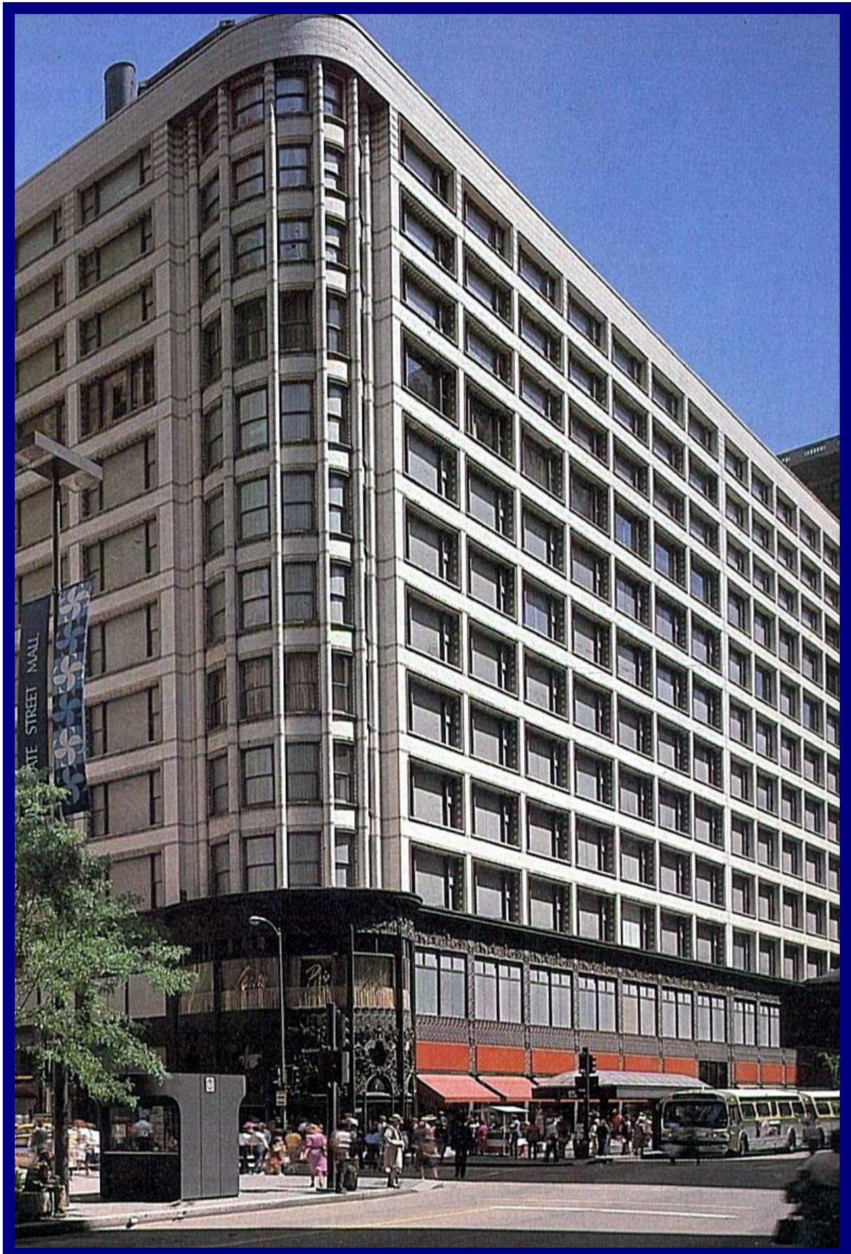
12 floors. Steel-framed fireproof structure.
