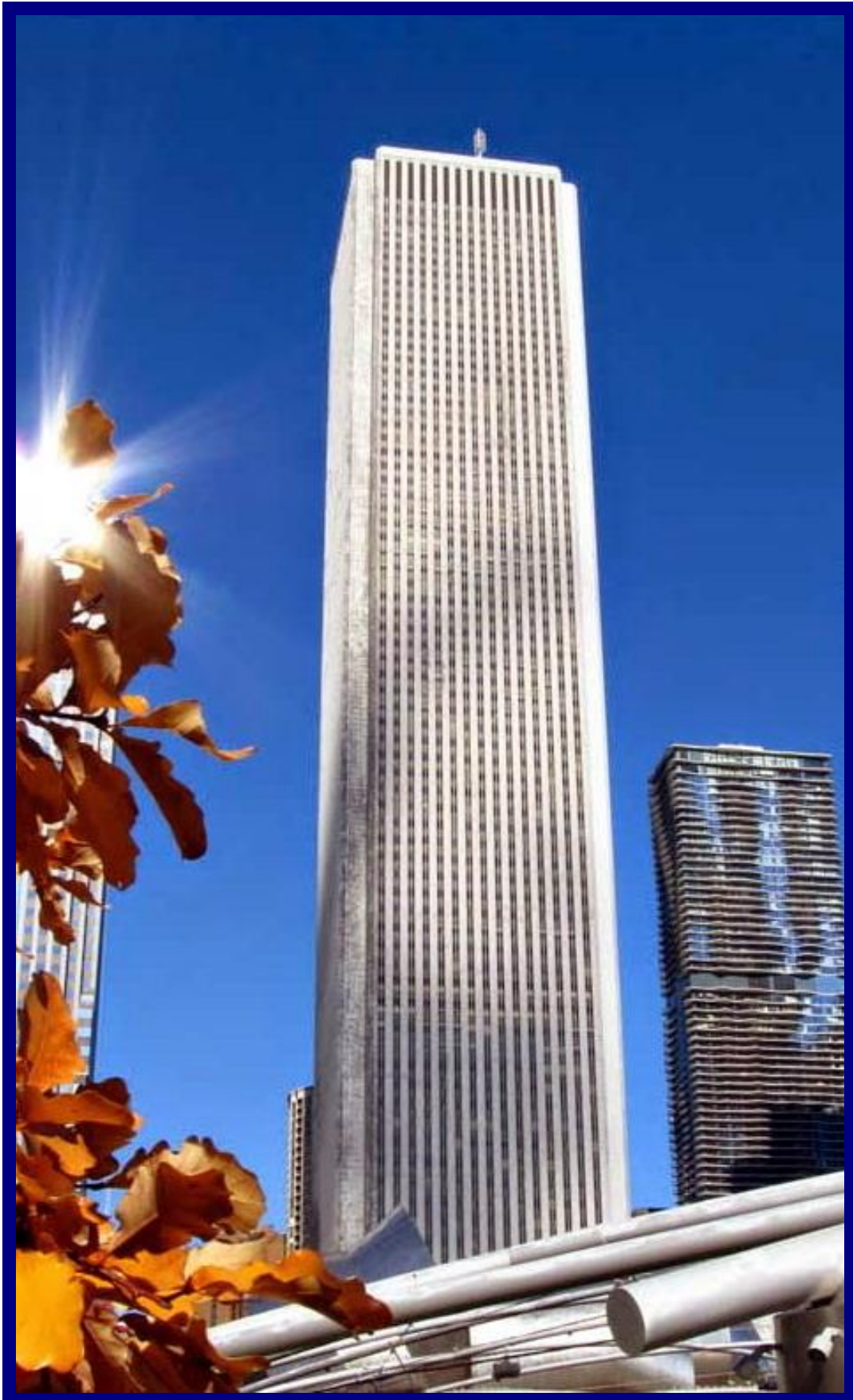
83 floors, 1136 ft. Architect: Edward Durell Stone. Renamed Amoco, then Aon Centre. The complete marble sheathing replaced by granite slabs after problems.
