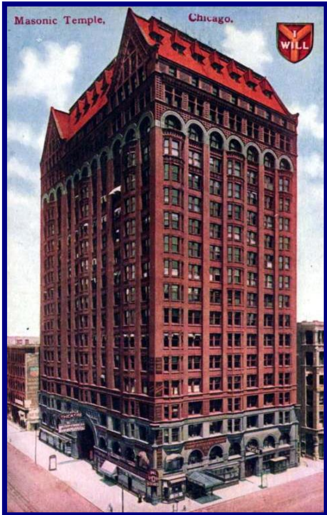
21 floors, 302 ft. Architect: Burnham & Root. Demolished 1919 (elevators proved inadequate).
