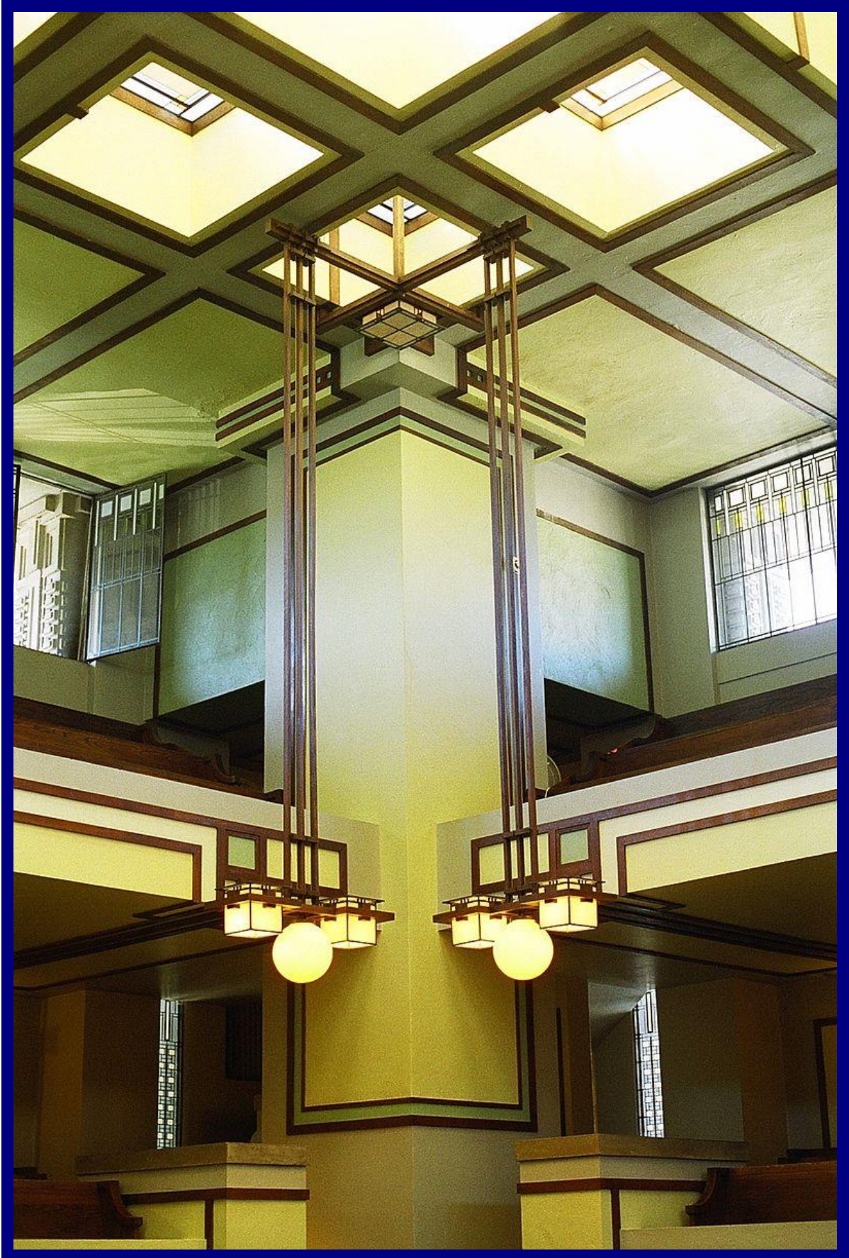
Has top-lit natural lighting through stained glass windows in roof and clerestories.
