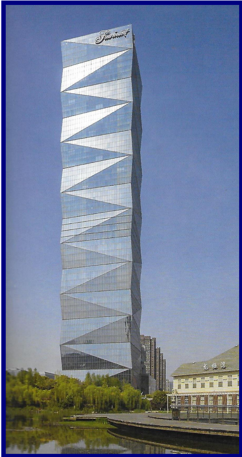
Hotel (Fairmont), 56 floors, 761 ft. MEP engineer WSP. 20 elevators.
