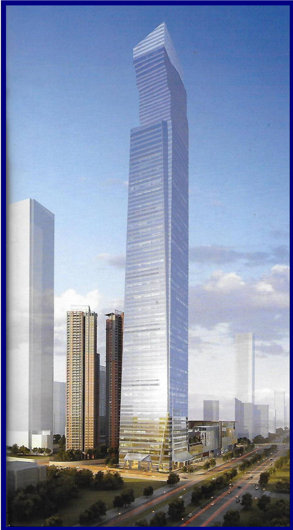
Offices & Hotel, 89 floors, 1321 ft. MEP engineer Parsons Brinckerhoff.
