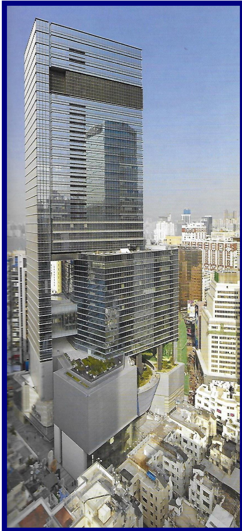
Office & Retail, 36 floors, 669 ft. MEP engineer Parsons Brinckerhoff.
