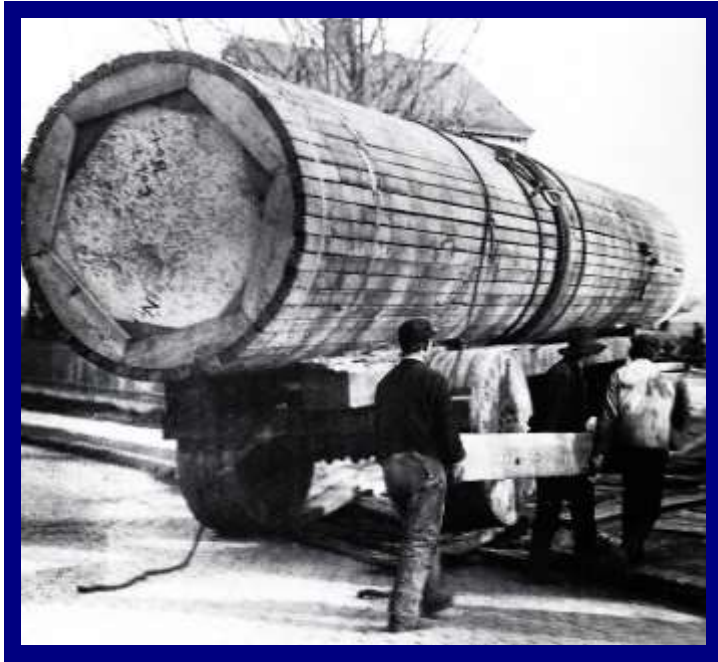
Taking a column to site 1904.
