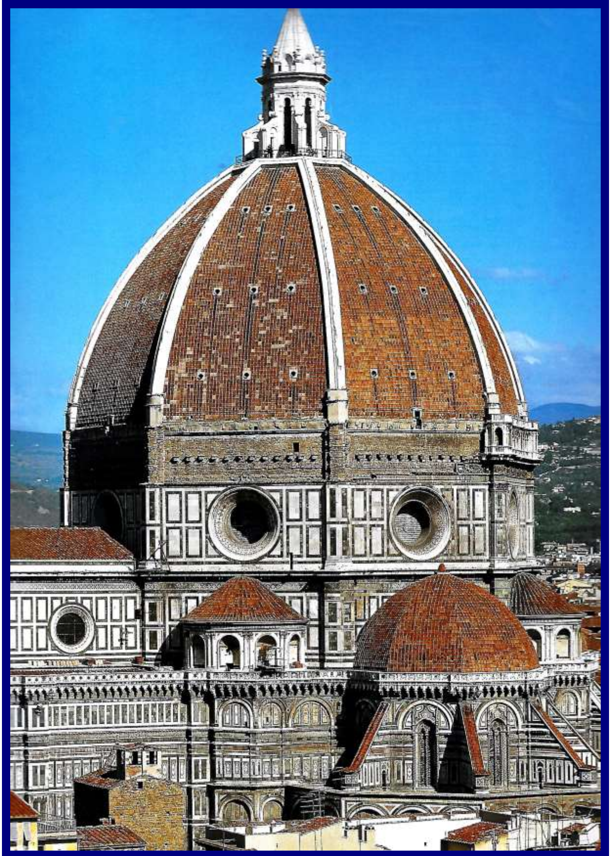
Built 1436, having largest brick dome ever constructed, employing a double-shell design.
