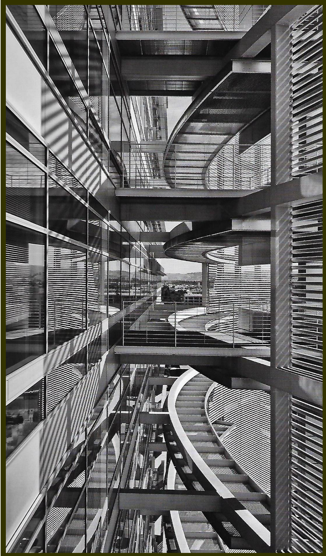
The brise-soleil shielding the 18-storey office tower and improving energy-efficiency.
