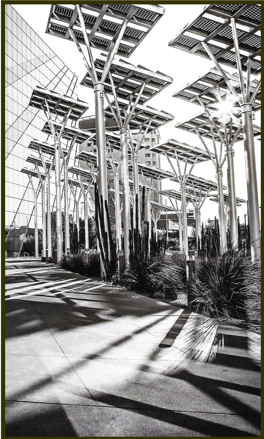
The forest of photovoltaic "trees" collecting solar energy.
