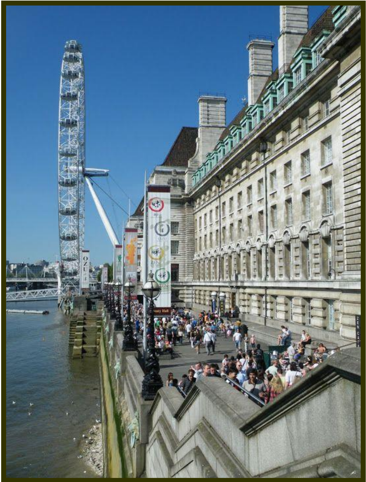
Heating and Ventilation by J. Jeffreys leading a consortium of Crittall, Haden, Norris & Dutton. Council Chamber air conditioning by Buffalo Forge and Carrier.
