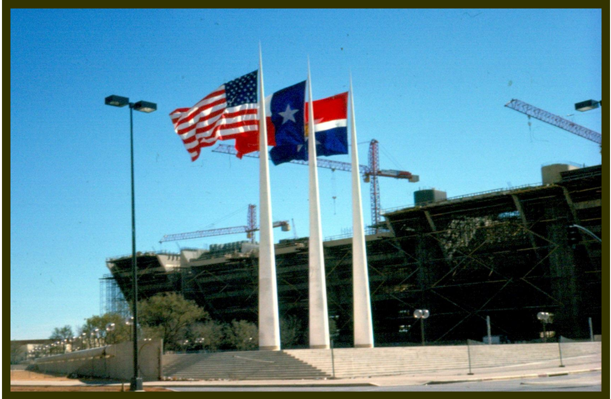
DALLAS CITY HALL under construction (author's photo)
