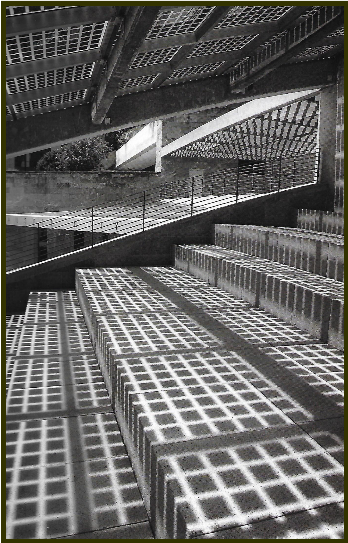
A photovoltaic glass trellis provides 10% of the Hall's power.
