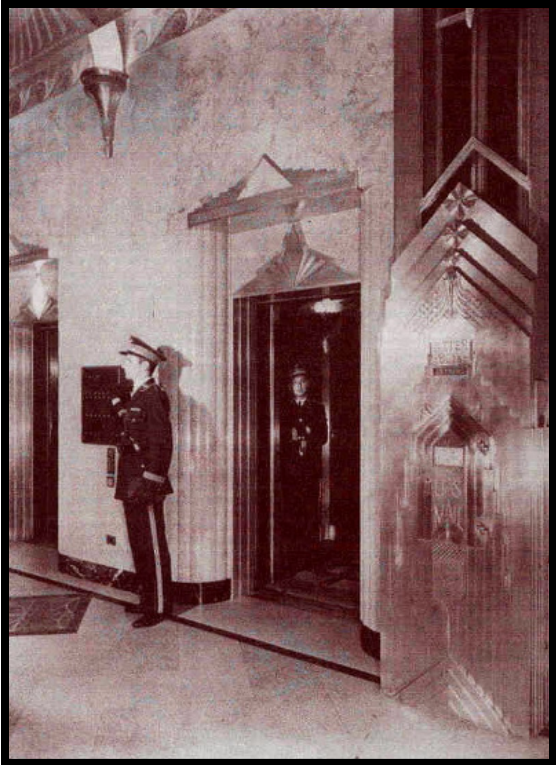
Lift lobby. Building opened 1933, 850 ft tall, 66 floors with 60 elevators.
