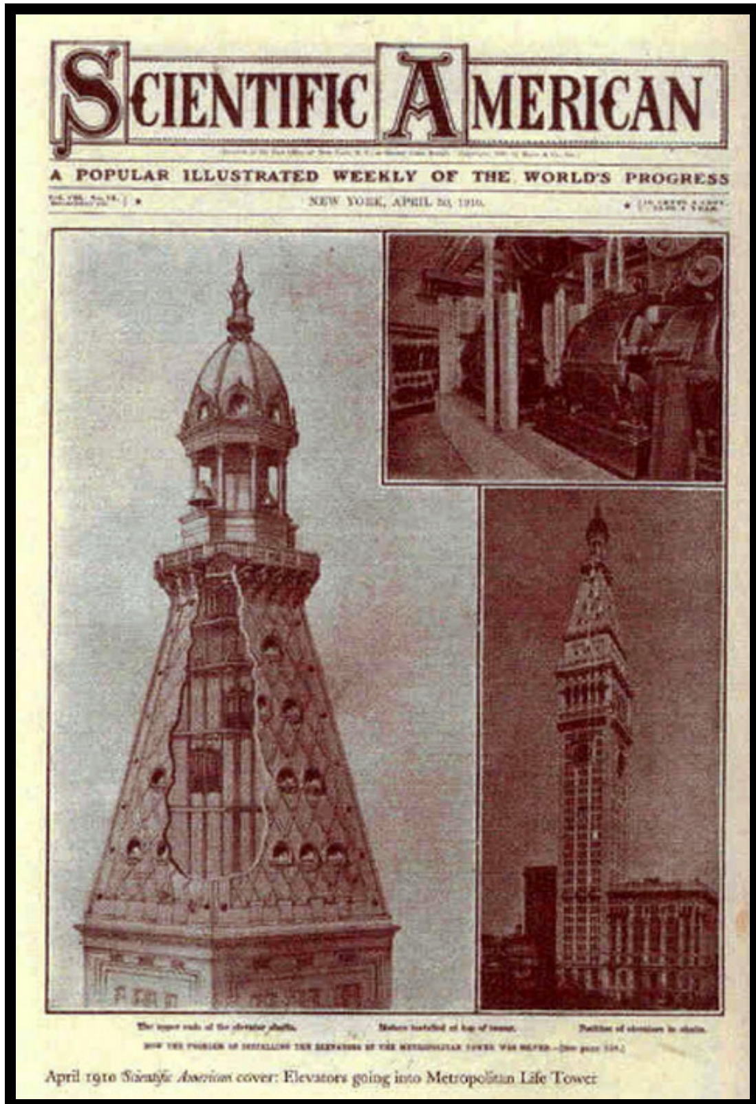
700 ft high, 50 floors. Elevators being installed 1910.
