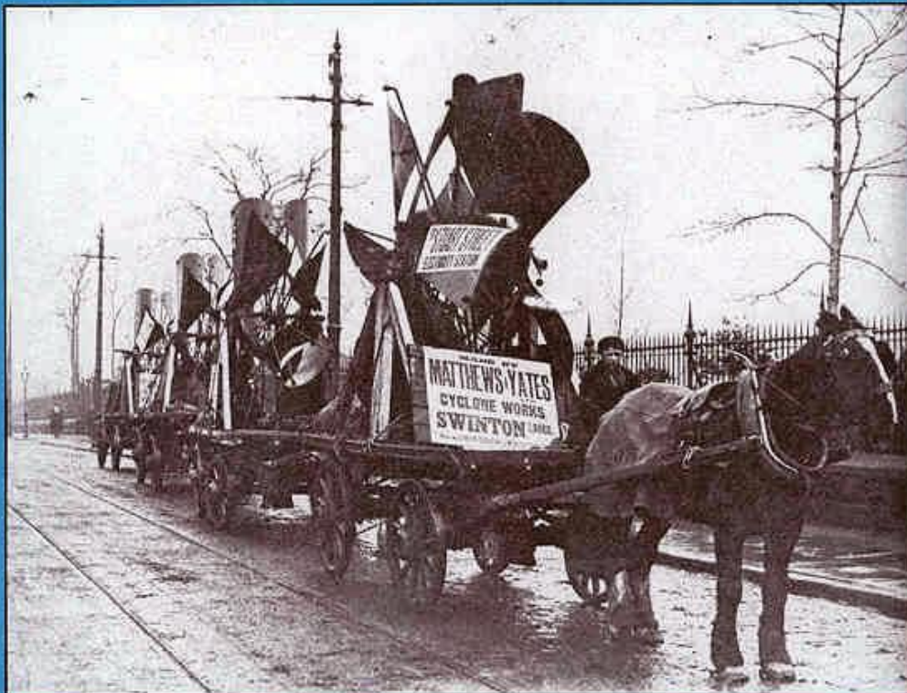
Delivery of M&Y Fans from Swinton, Manchester to Stuart Street Electricity Station, 1890s. [BSE, 1, 45, April 1977]
