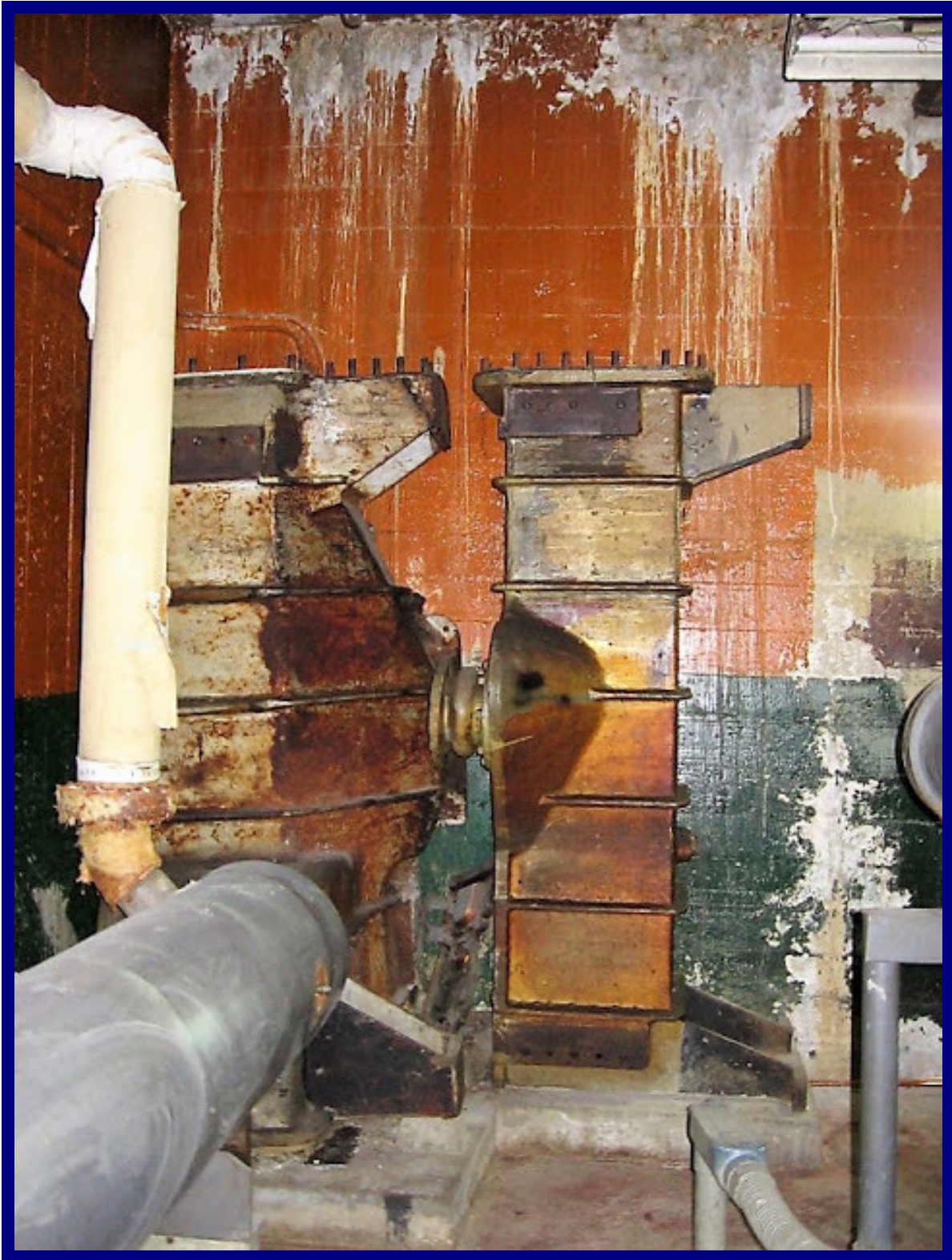
Remains of the 1927 air conditioning system
