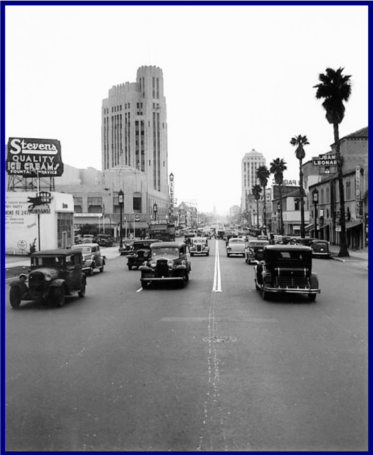
Wiltern Theatre (once Warner Theatre) in the mid-1930s. Opened 1931, 1850 seats. Originally evaporative spray washer cooling system, refrigeration added in 1984
