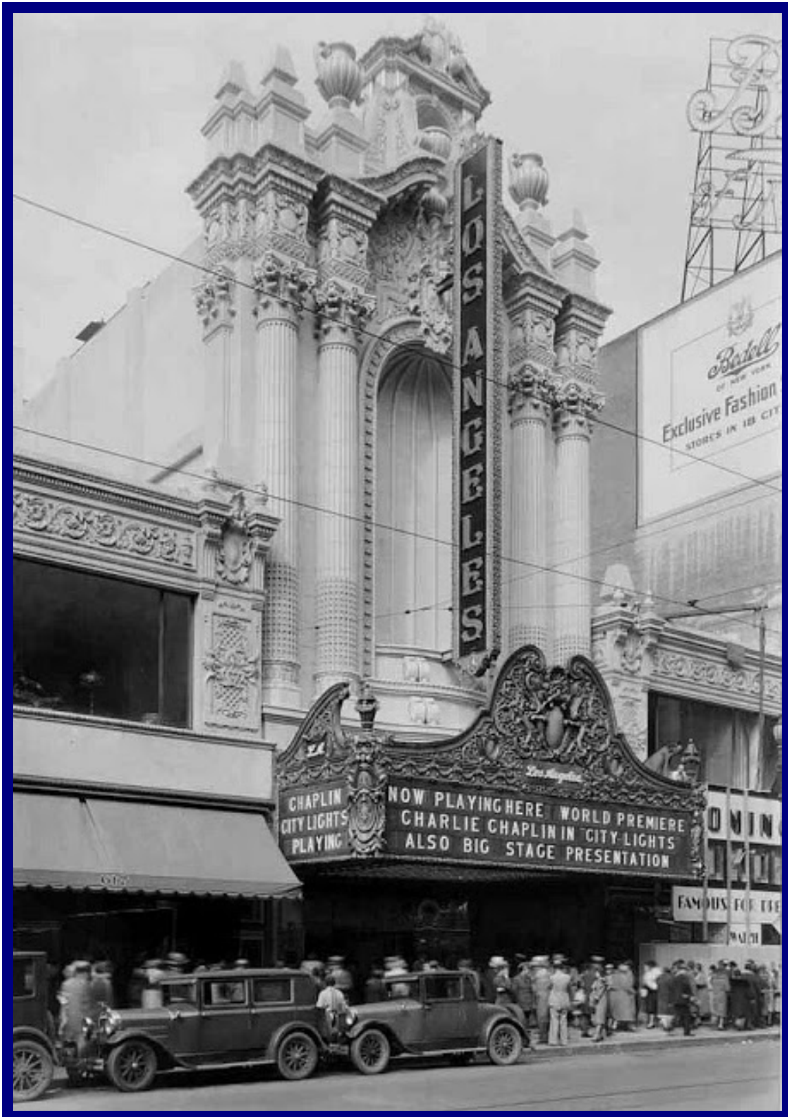
Los Angeles theatre in 1931. Opened 1927, 2190 seats Air conditioning by Carrier
