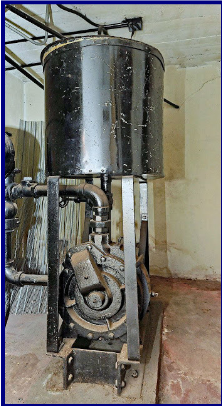
Hydraulic mechanism for organ lift
