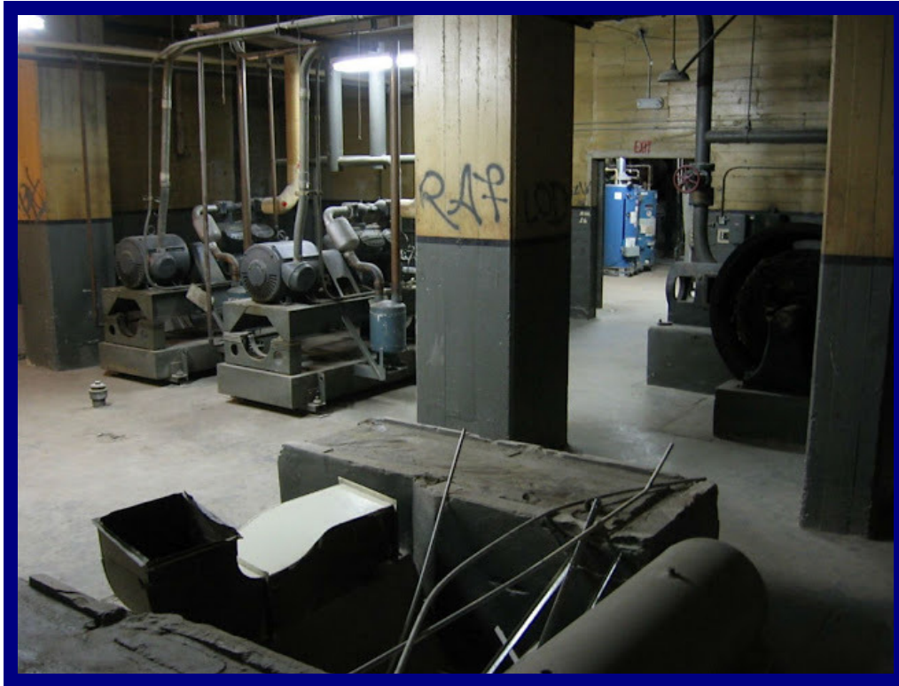
Refrigeration compressors
