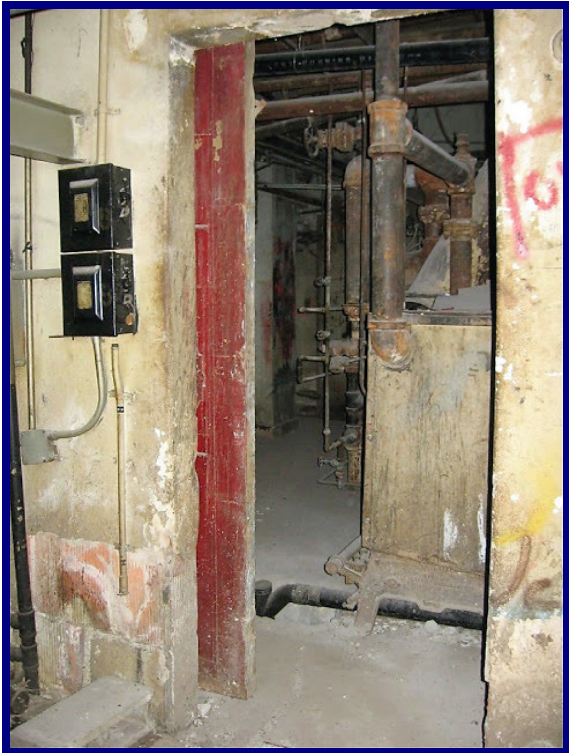
Looking into the boiler room
