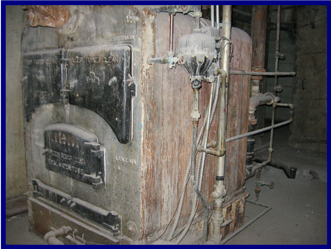
In the boiler room
