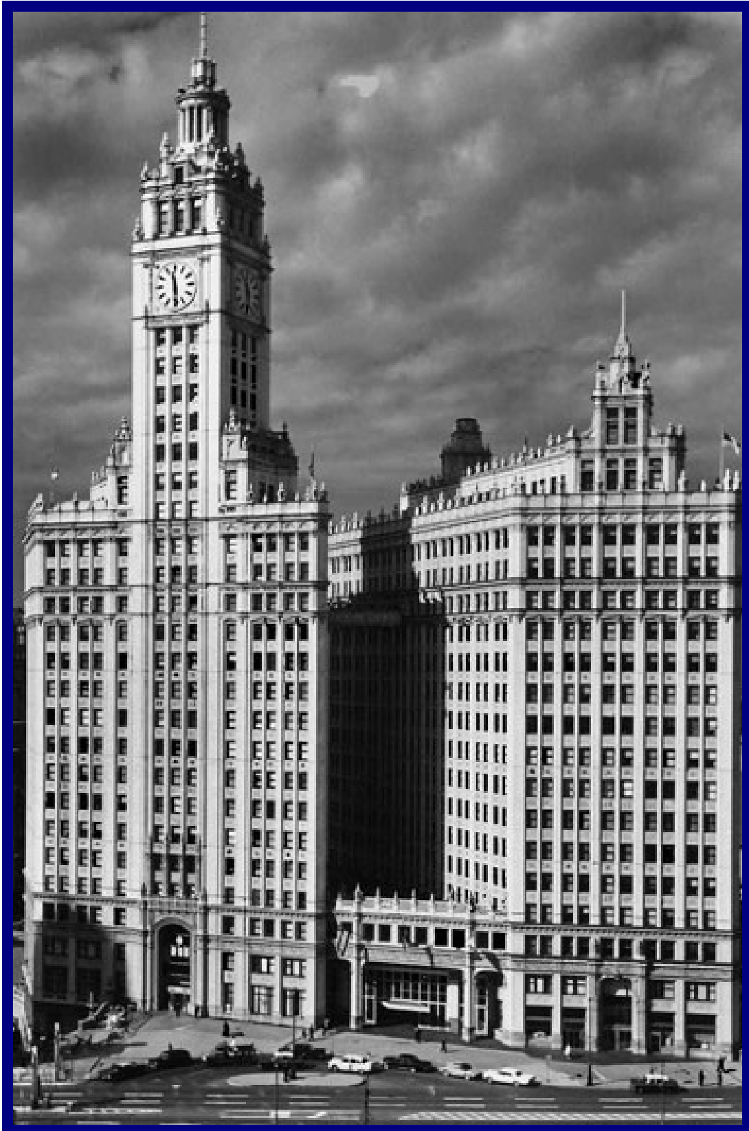
1924: 438 ft (spire), 30 floors (North Tower), 21 floors (South Tower). Architect: Graham, Anderson, Probst & White. Air conditioning in a few areas, Wittenmeier Machine Company (1927 advert). Possibly CO 2 refrigeration.
