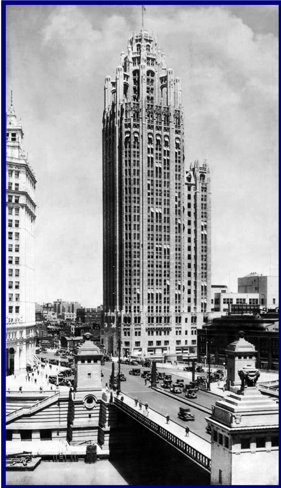
1925: 462 ft, 34 floors. Architect: John M. Howells & Raymond Hood. Air conditioning in a few areas. Wittenmeier Machine (1927 advert). Possibly CO 2 refrigeration.
