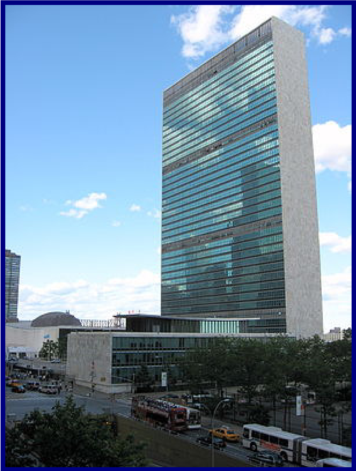
1951: 510 ft, 39 floors. Architect: Oscar Niemeyer, Le Corbusier, Wallace Harrison. Air conditioned by Carrier Weathermaster induction unit system (Ingels, p.95).
