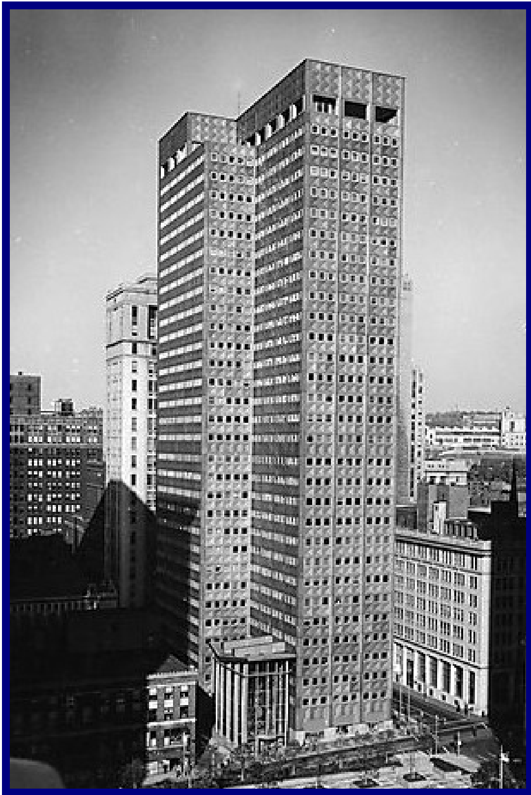
1953: 410 ft, 30 floors. Architect: Harrison and Abramovitz. External wall cladding is thin lightweight aluminium. Offices provided with radiant ceiling panel heating and cooling systems.
