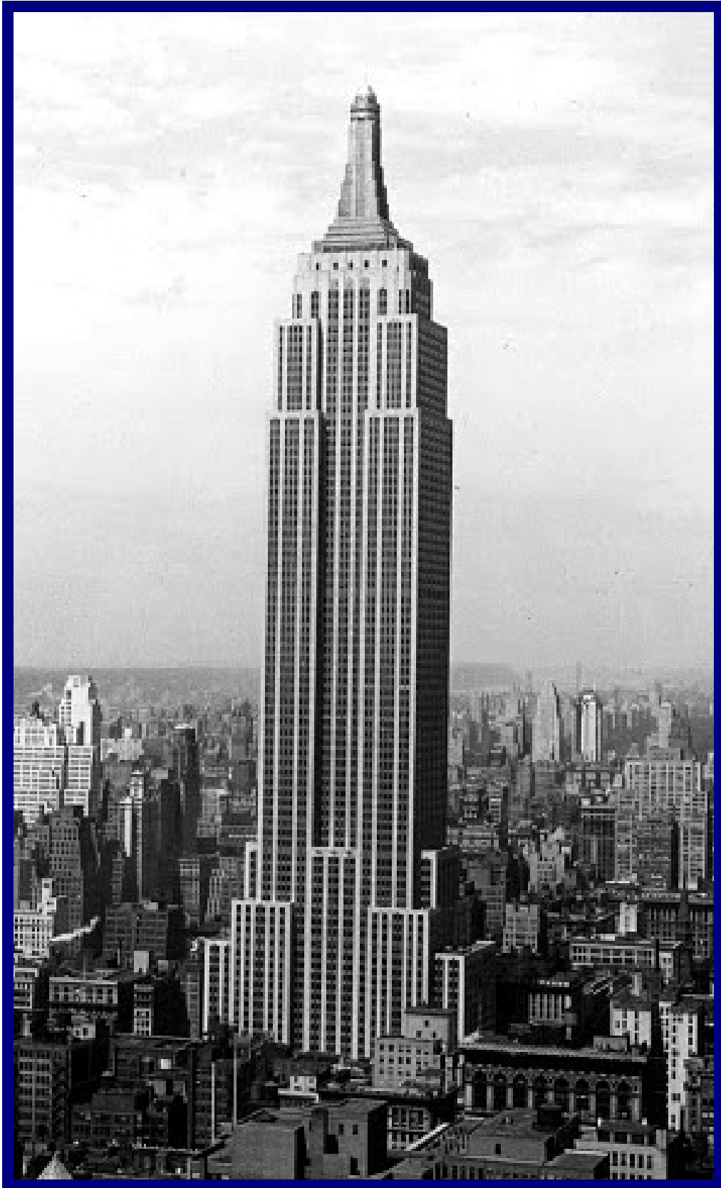
1930: 1250 ft, 102 floors. Architect: Shreve, Lamb & Harmon. Tallest building in the world 1931-1972. Not originally air conditioned. Air conditioning progressively added from 1950s.
