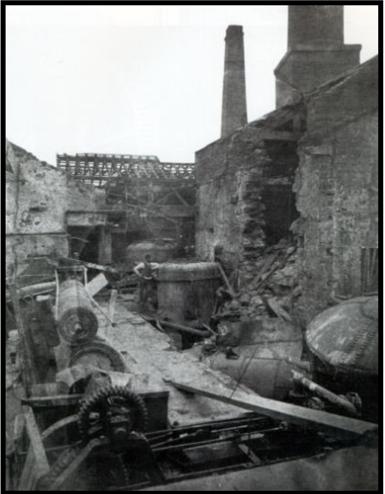
Aftermath of Boiler Explosion at Rose Bank Bleach Works, Ramsbottom, Lancashire, 1873.
