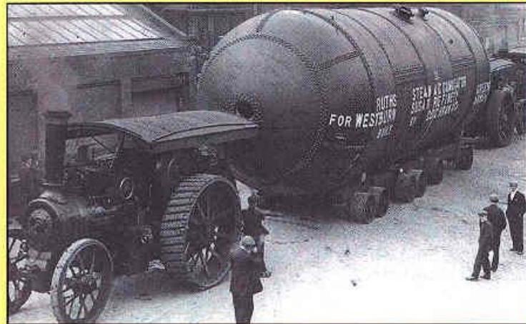
Ruth's Steam Accumulator made by Cochran for Westburn Sugar Refinery, c.1930
