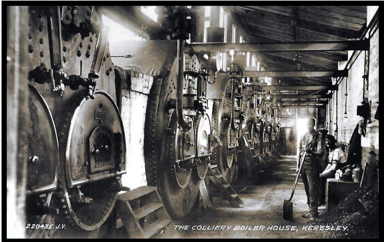
Boiler House at Keresley Colliery, near Coventry.
