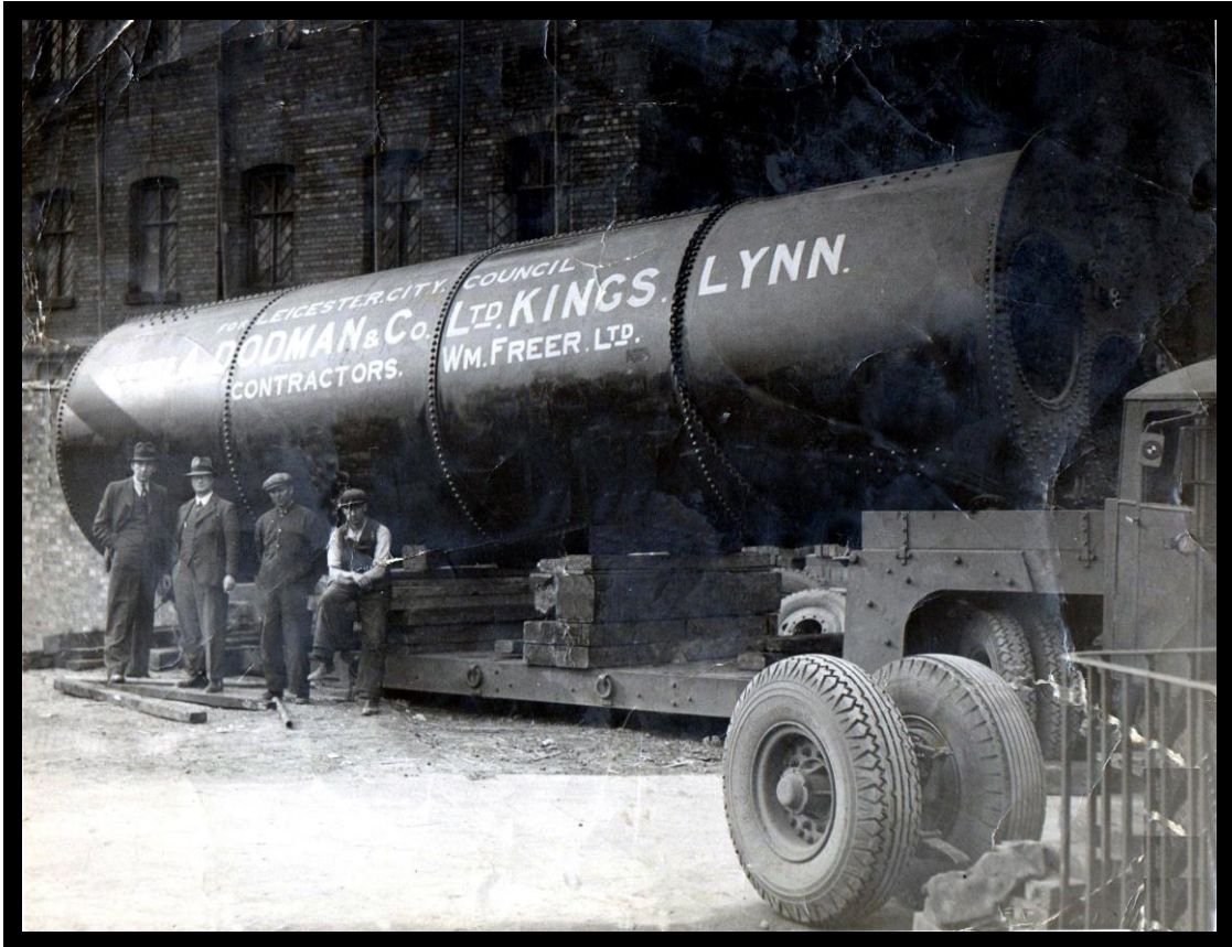
Transporting a Boiler for Contractor Wm. Freer Ltd of Leicester.
