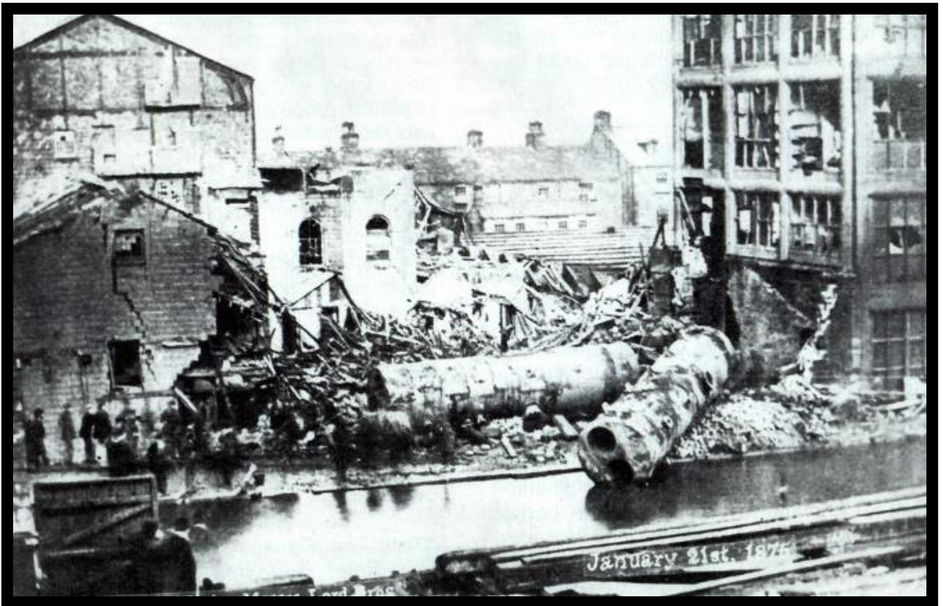
After the Boiler Explosion at Lord Brothers, Todmorden, West Ridng of Yorkshire, 1875.
