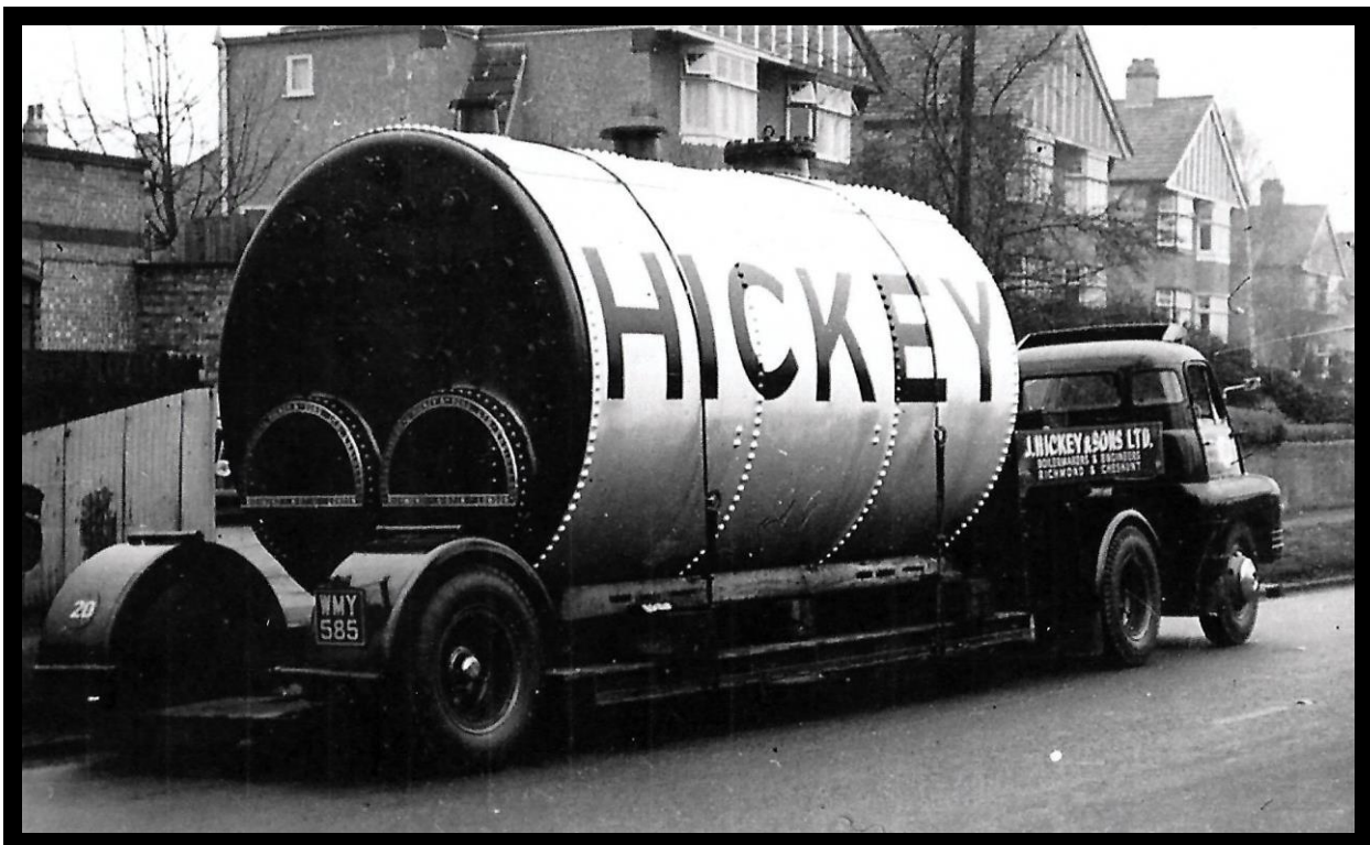
Boiler by J. Hickey & Sons Ltd, Richmond.
