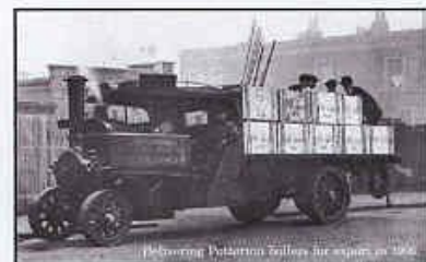
Delivery of Potterton boilers, 1906
