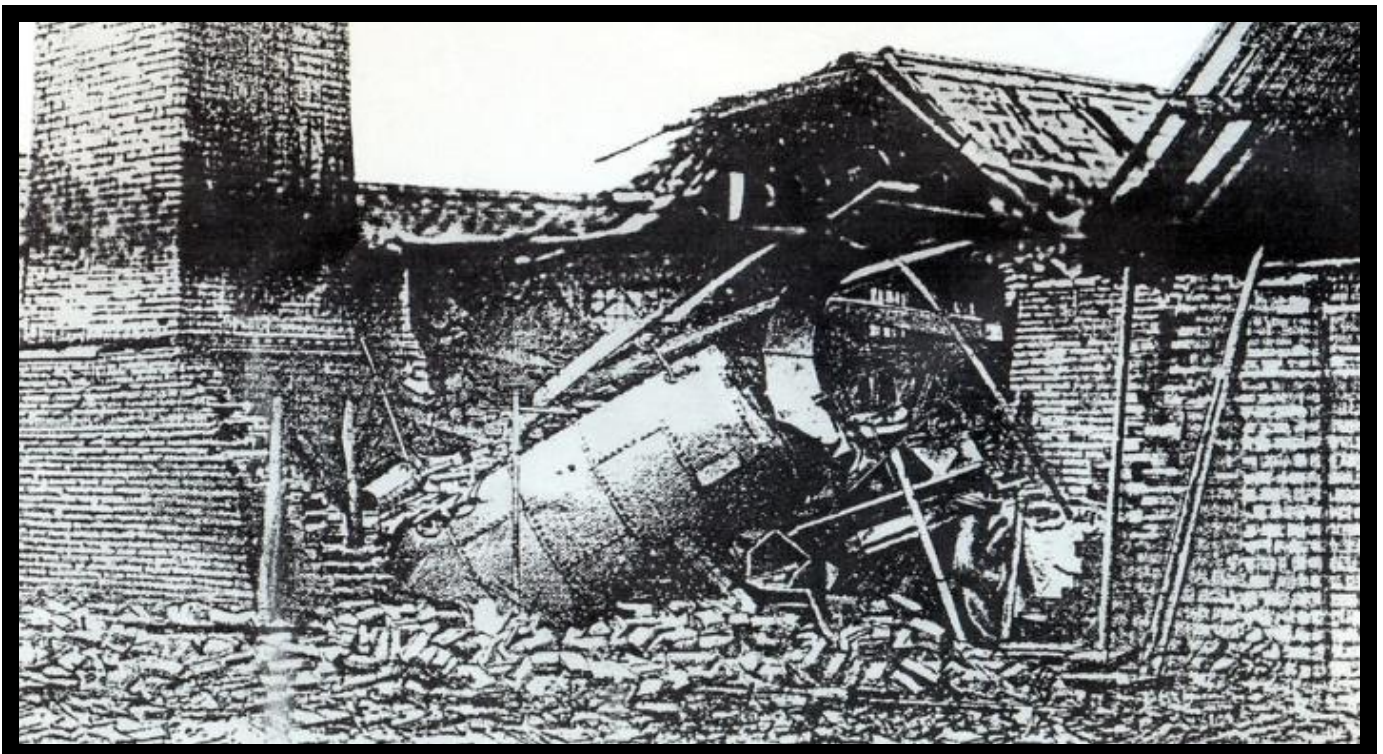
Destruction of Egg-Ended Boiler and Building at Bridgefield Mill, Rochdale, 1854.
