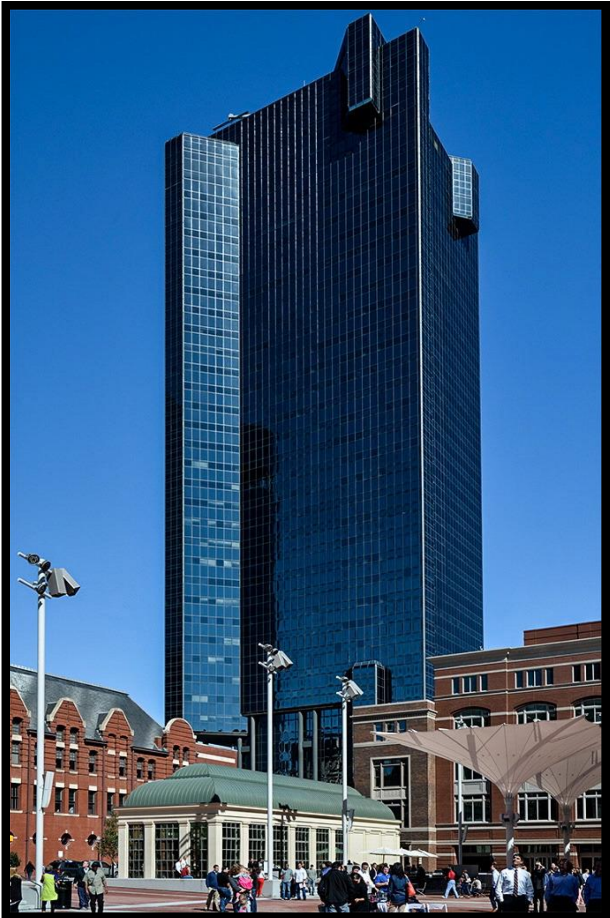
1984, 547 ft, 38 floors. Look-alike design to Wells Fargo Tower (p.39).
